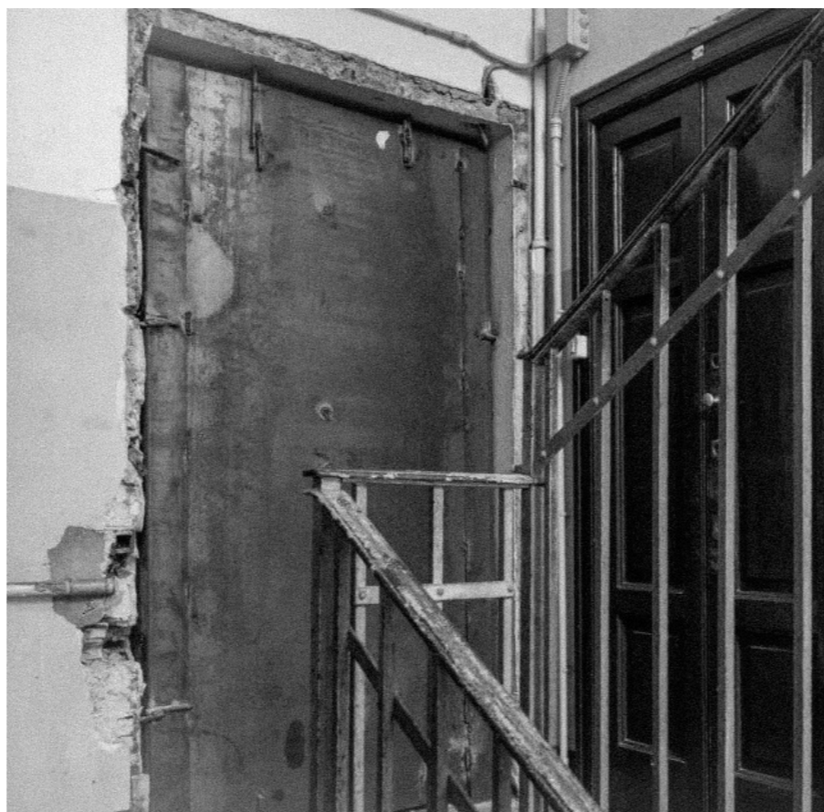
↑ The accommodations empty is also locked with heavy plates of iron, which, however, are often torn.
