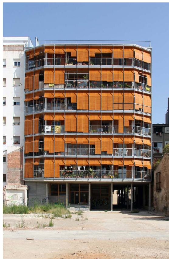
P1. External view of the building
