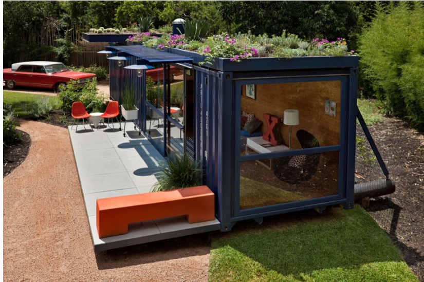
Figure 22, Container guest house by Poteet Archietctcs
