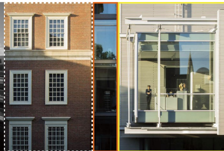
Fig. 22 Museum South Facade Part 21
