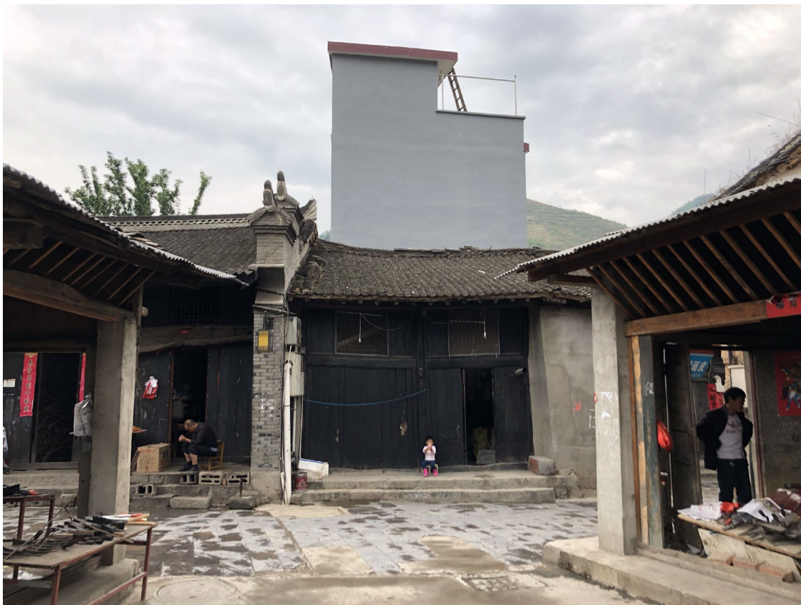
Fig. 80 Concrete replacement of old block
