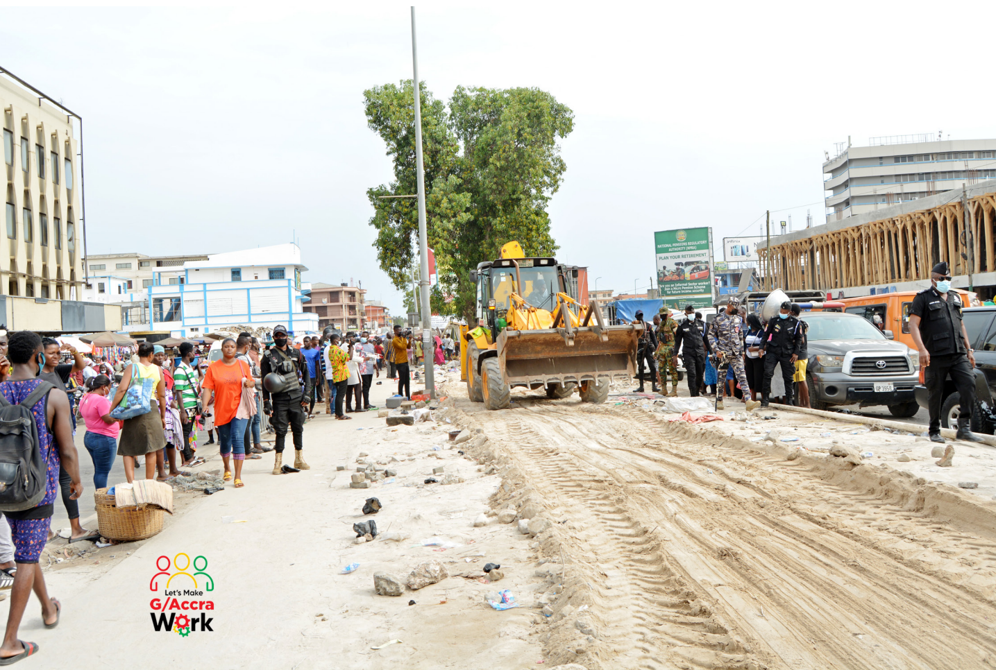
Figure 5.2: Ongoing decongestion activities in Accra
