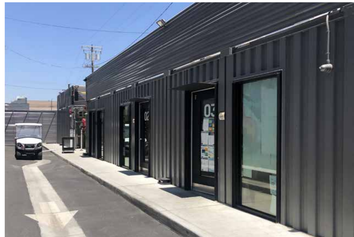
Rows of shipping containers used to create Ghost Kitchen for delivery only, Los Angeles
