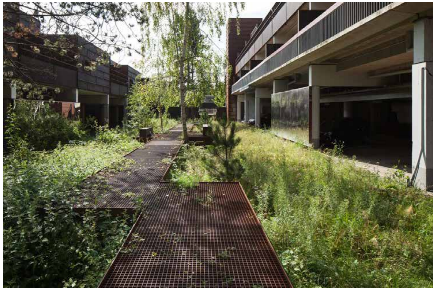
Case study of a steel grating walkway
