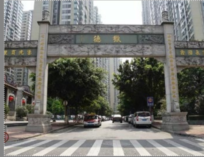
Figure 2.22 The complete rebuild of Liede Village
