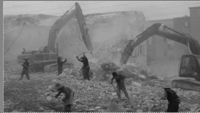
Figure 2.1 Demolishing urban villages
