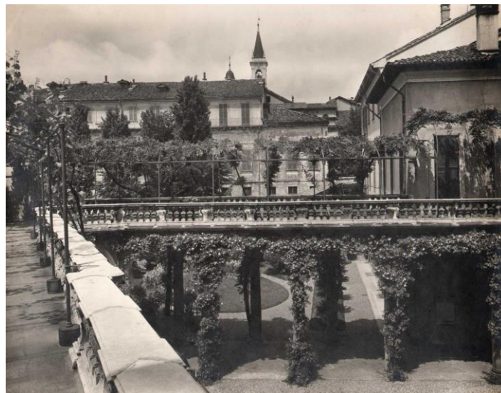
Figure 42. View of the courtyards of Palazzo Archinto , 1934
