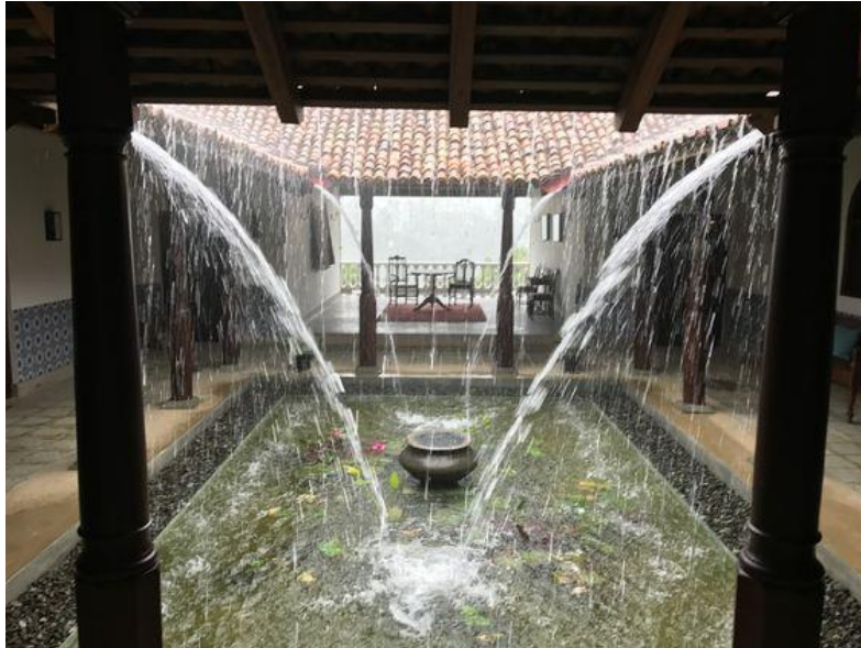
Figure 37. A Chettinad courtyard used for rainwater harvesting and sustainable practices.
