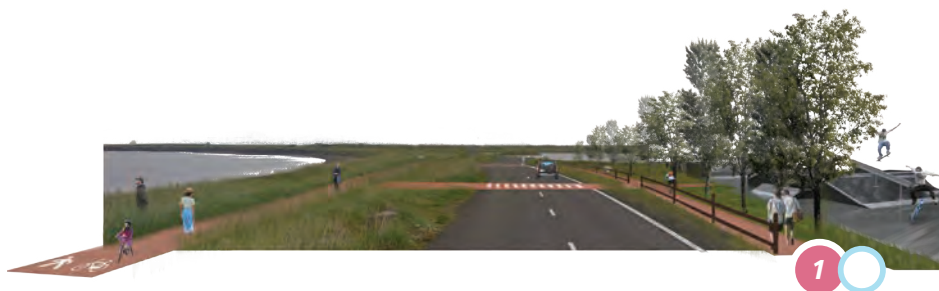
Figure 127: Transformation on Sudurstrond Street, Zone 1.
