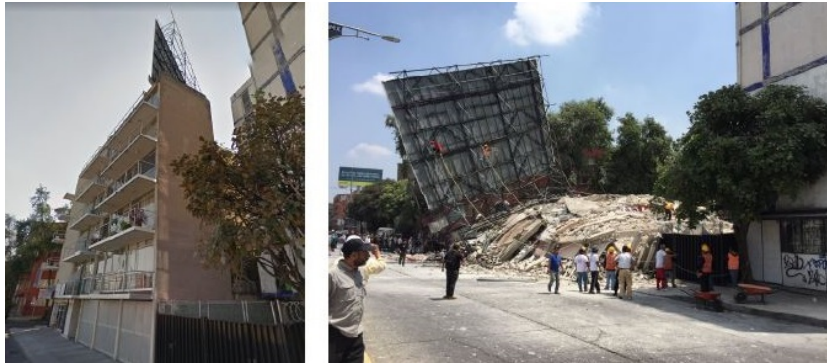
Figure 2.42: Collapsed building with flat slab system at Viaducto Miguel Alemán 106, Piedad-Narvarte, before the 2017 Puebla-Morelos earthquake (left) and after the earthquake (right). [From Galvis et al. (2017)].
