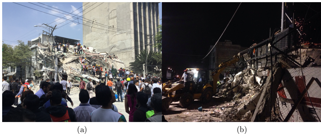
Figure 2.8: Collapsed buildings in Mexico City after the September 19, 2017 earthquake. a) Building at Medellin 176 b) Building at Simon Bolívar 190. [Source:ProtoplasmaKid/WikimediaCommons /CC-BY-SA4.0].
