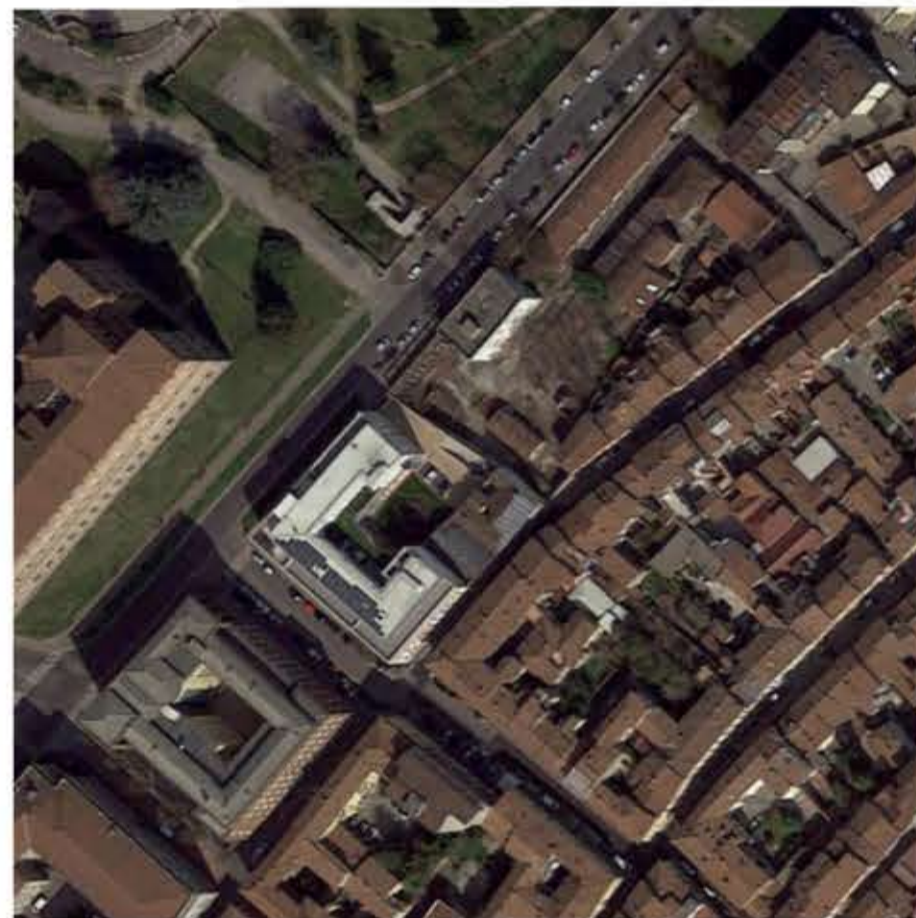
Existing friendly, pedestrian oriented, paved road Via Bacciochi.
