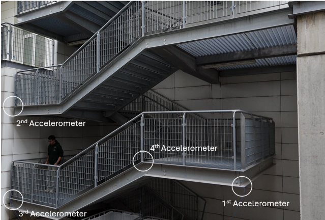
Figure 4: Laboratory-area staircase with accelerometer locations.
