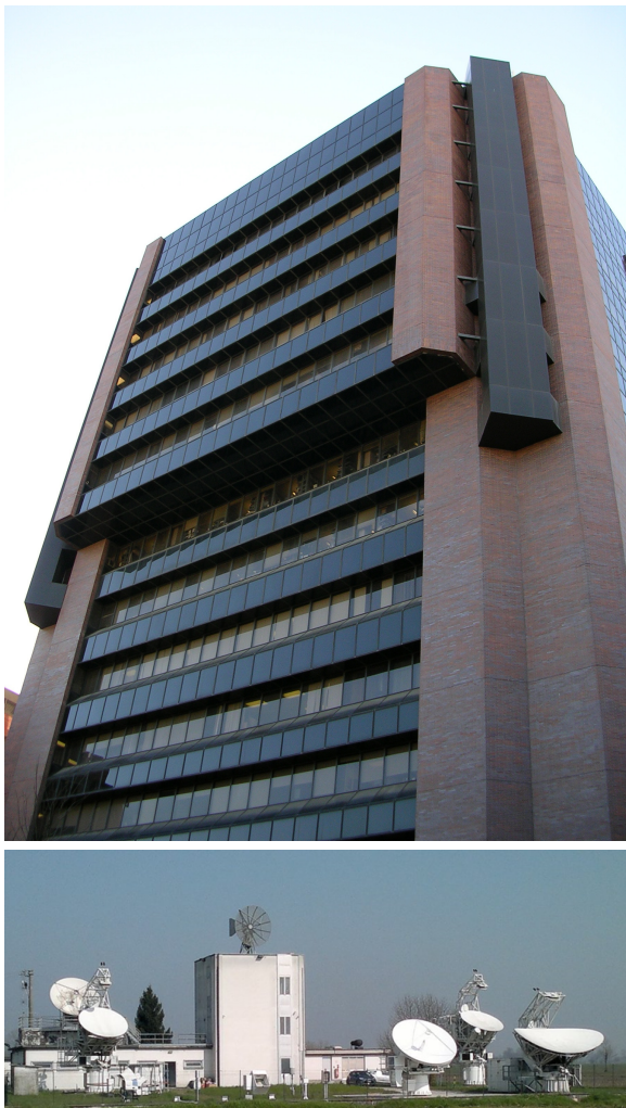
Figure 2.1: Buildings used in our tests. From the top: University of California, Los Angeles building, and the meteorological station in Spino d'Adda, Cremona, Italy.
