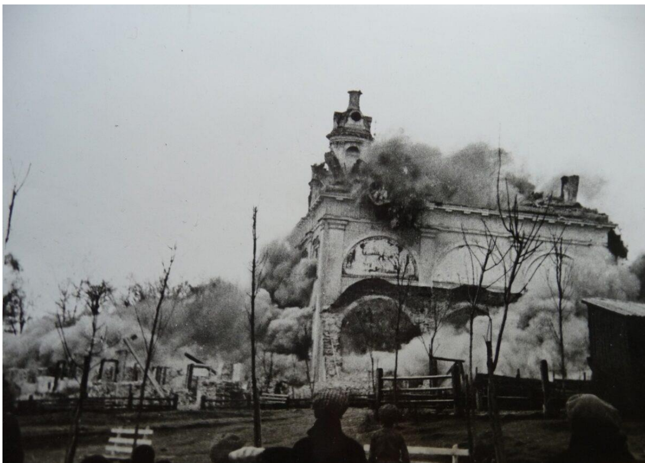
Figure 6 The explosion of Pokrovsky Cathedral in Kimry, 1936. Photo: PANORAMA Pro
