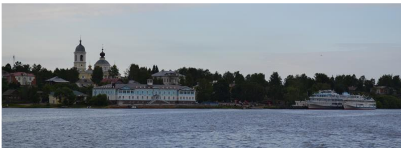
Figure 18 Myshkin embankment in 2015
