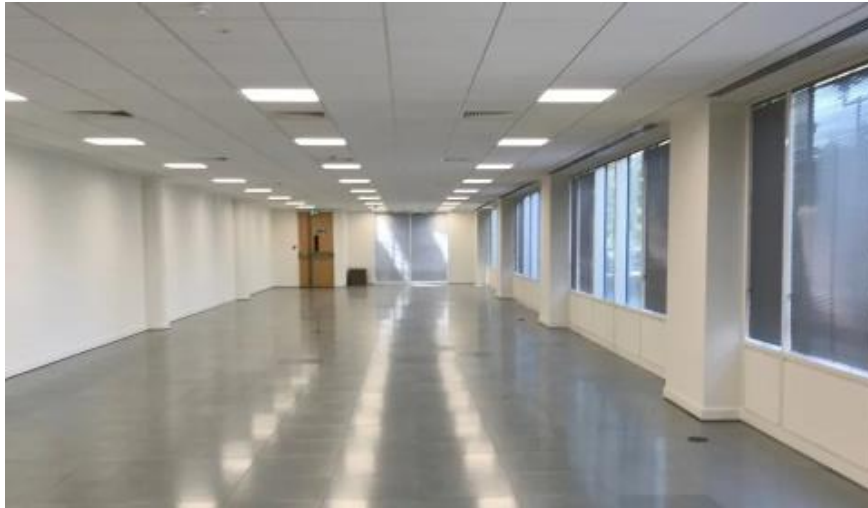
Figure 26 - Example of Cat A fit-out (source: RAP interiors)
