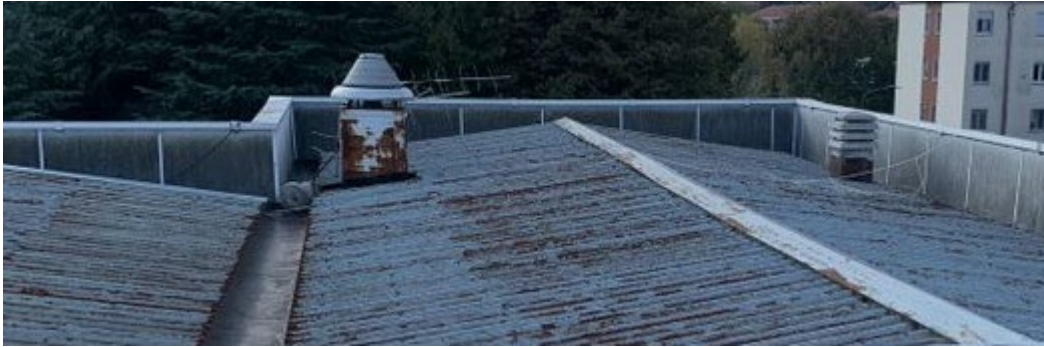
Figure 10 - Picture of the roof
