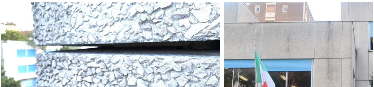
Figure 9 - External wall pictures
