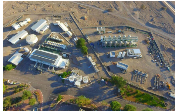
Figure 8. Eilat's desalination. Source: Mekorot
