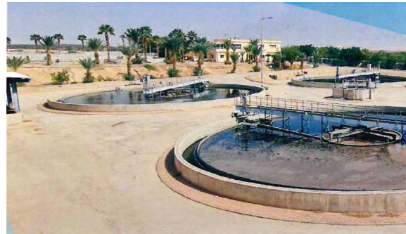
Figure 7. Eilat's desalination. Source: Mekorot
