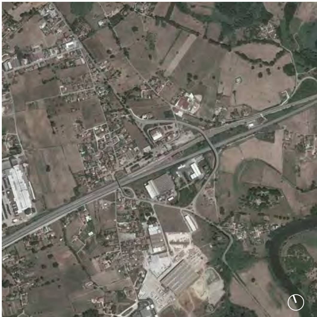
Fig. 198 Satellite view of the Ceprano station
