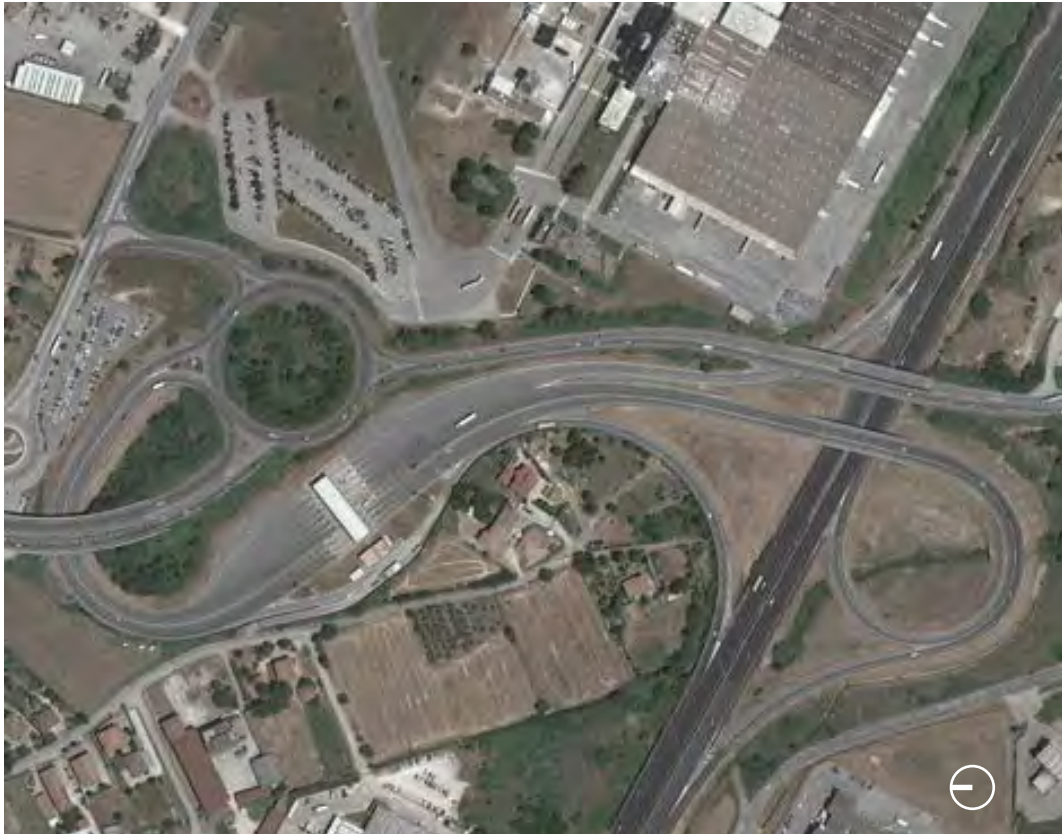
Fig. 108 The Ferentino motorway toll booth
