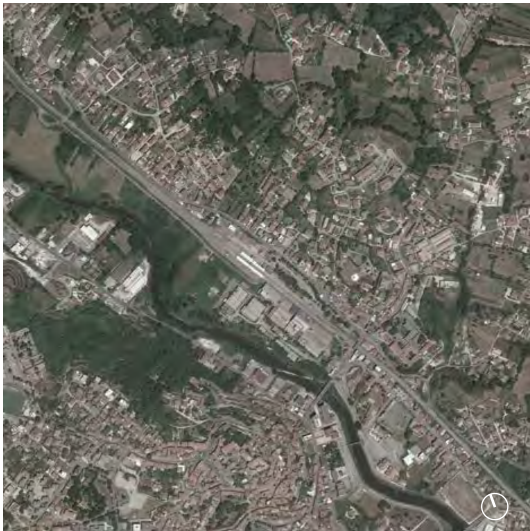
Fig. 184 Satellite view of the Colleferro station
