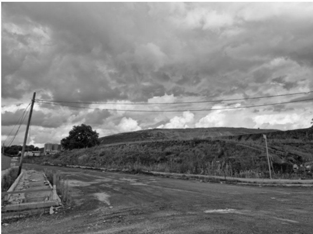
Fig. 115 The closed landfill
