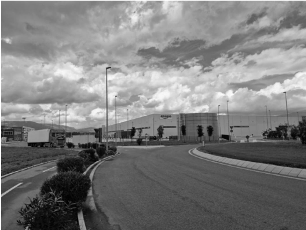
Fig. 112 The new Amazon warehouse
