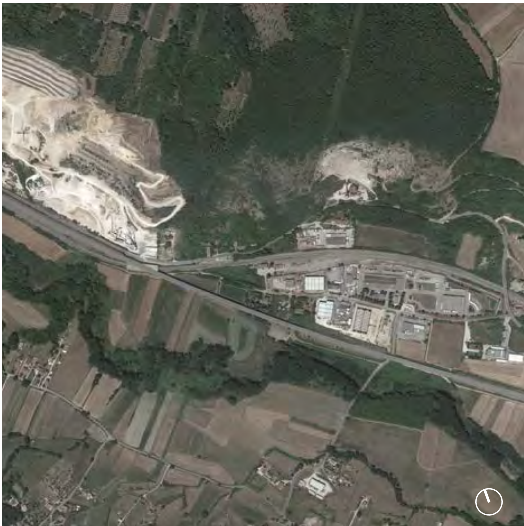
Fig. 171 Satellite view of the Morolo station
