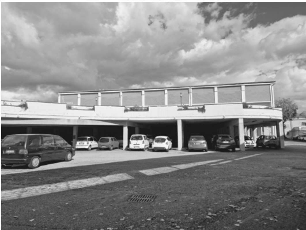
Fig. 159 The multilevel car parking and the auditorium
