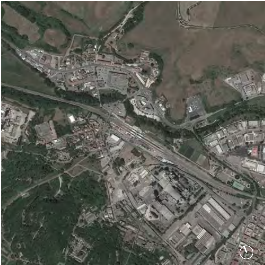
Fig. 154 Satellite view of the Colleferro station
