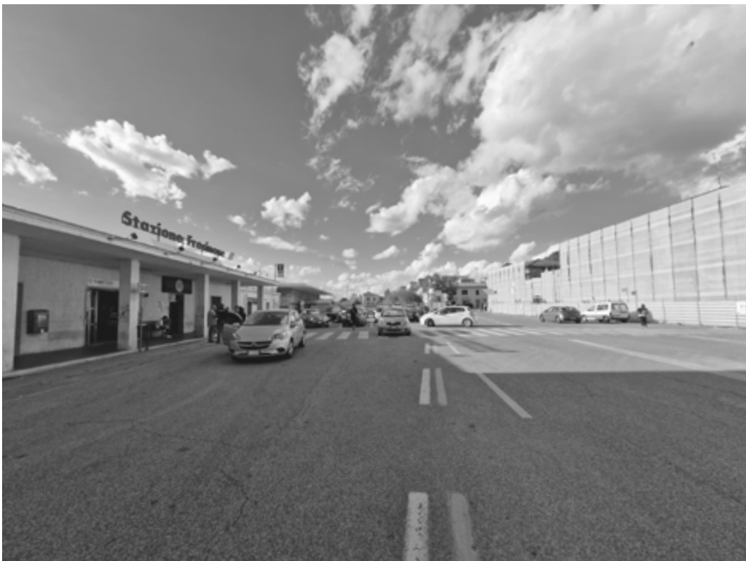
Fig. 180 The front square and the renovation works in progress
