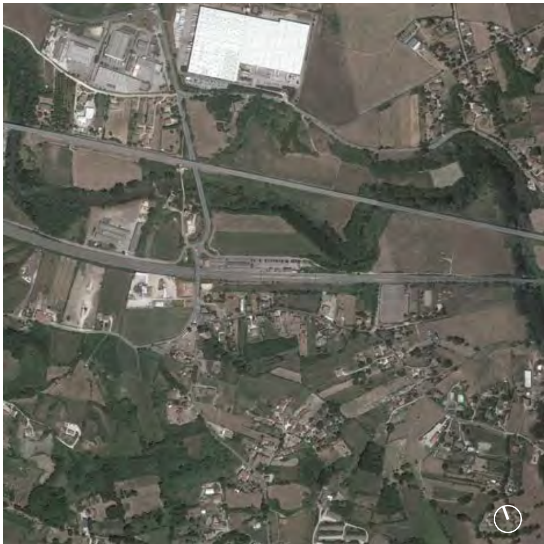
Fig. 168 Satellite view of the Sgurgola station
