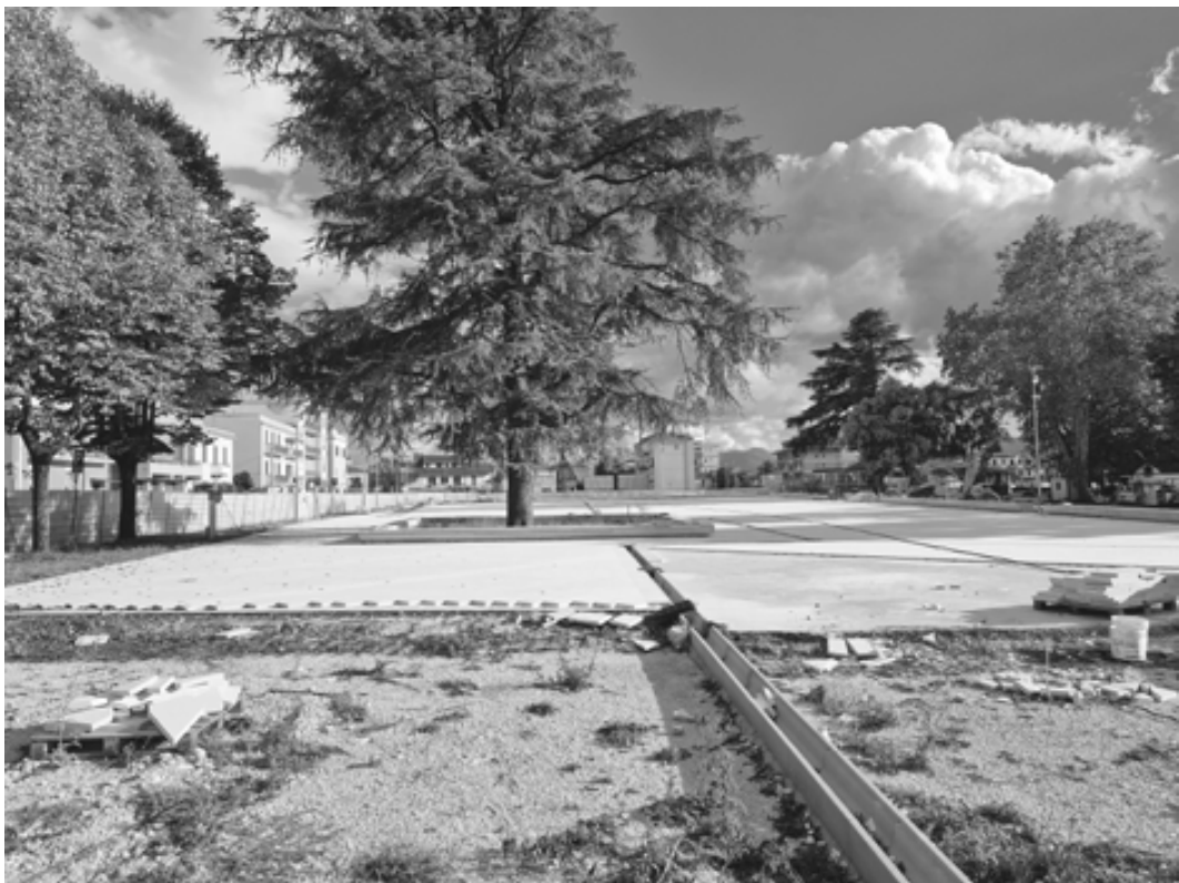
Fig. 182 Works in progress for the new square
