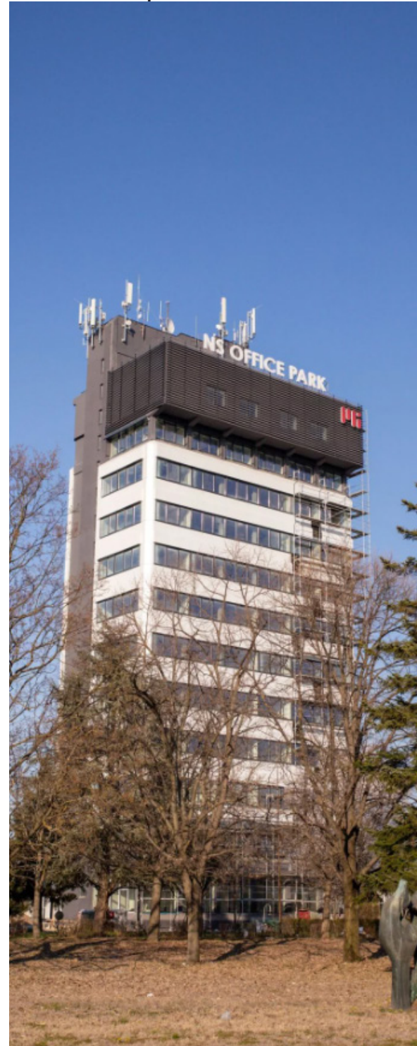
Figure 3.39 (left) Novkabel (computer and cable factory) tower before reconstruction (Source: Nevena Popovic)
