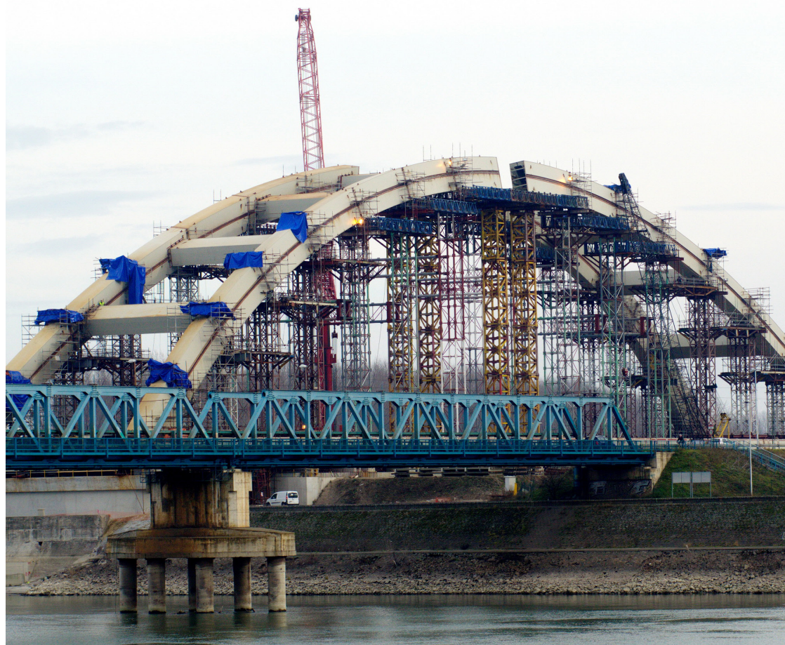
Figure 3.36 (left) Works on the construction of the Zezelj bridge. (Source: gradnja.rs)
