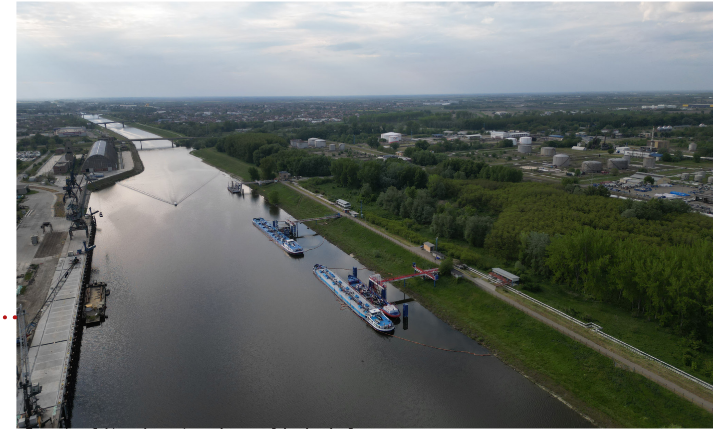
Expansion of shipyard capacity to the area of the closed refinery
