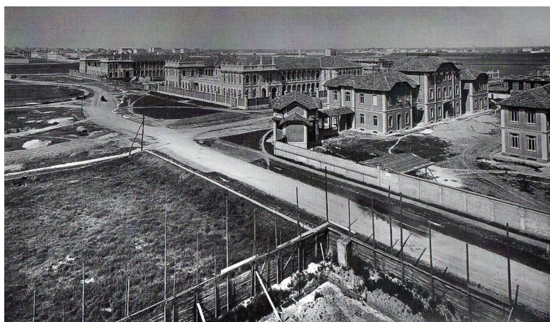
View of the Construction Site in 1924
