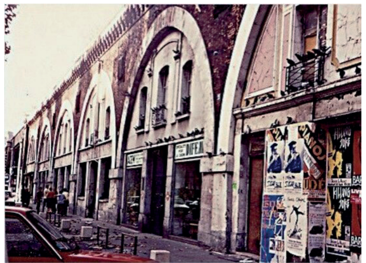
Figure 5. Gare de la Bastille shortly before its demolition.
