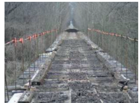
Figure 4. During construction of the greenline.
