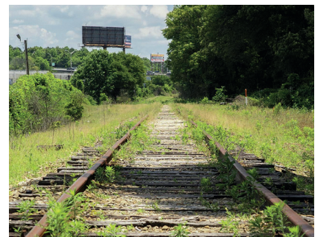
Figure 4. Rail tracks on site.
