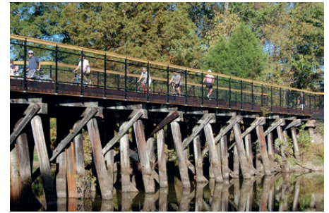
Figure 3. Historic railroad bridges of timber construction.
