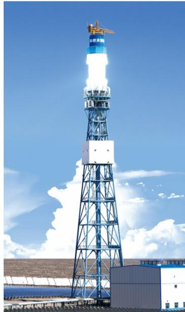
Figure 2.10: Steel lattice 80m tower in SUPCON Delingha 10 MW plant [32]
