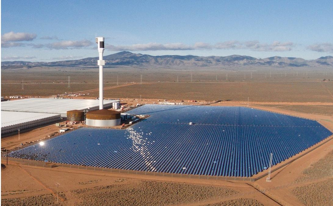
Figure 2.12: Steel monopole 127m tower in Sundrop plant [37]
