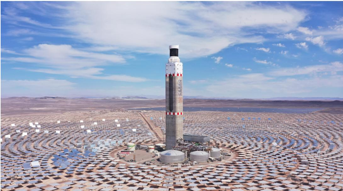
Figure 2.9: Concrete tower in the Cerro Dominador CSP plant, Chile [29]
