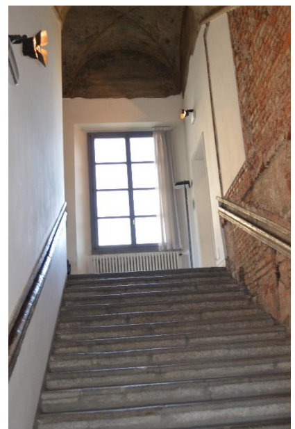
Figure 56: the main stair connecting floors of the building.
