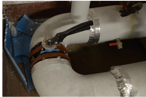
Figure 86: the valves that separate water outflows and inflows in the distributing system
