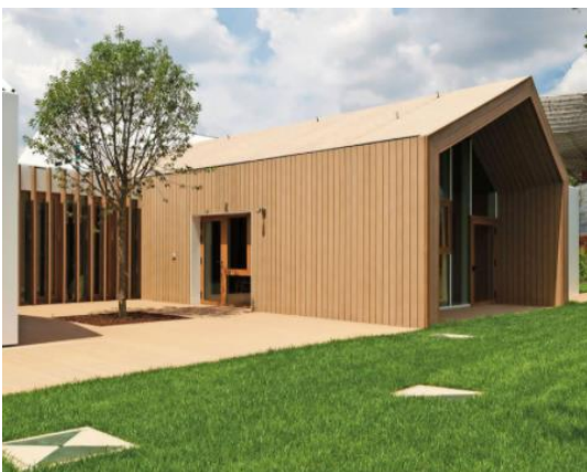
Figure 118: The wooden structure of Citylife Nursery School
