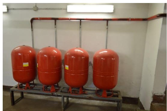
Figure 88 the expansion tanks to avoid excessive pressure inside the collecting tubes
