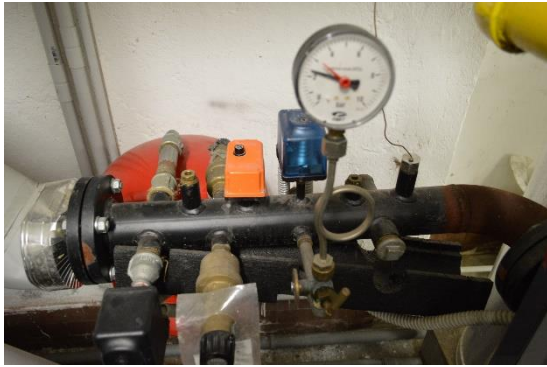
Figure 85: the system named “clarinetto” aimed at checking pressure and temperature of water before its introduction in the distributing system
