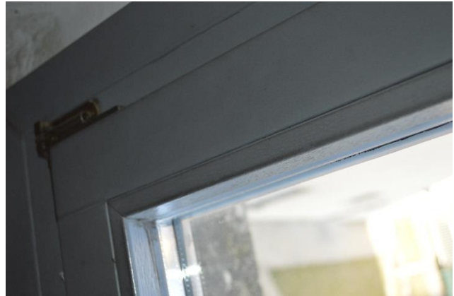
Figure 58 transparent surface is composed by 92 double glasses wood and aluminium window.
