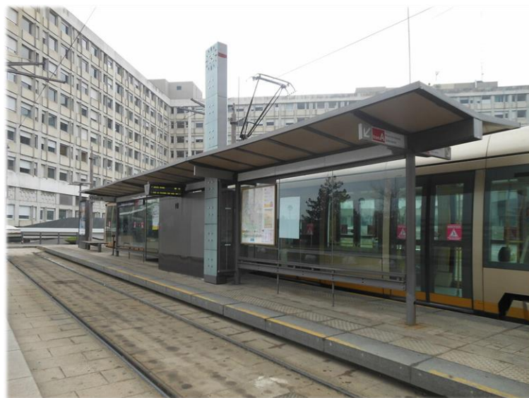
Figure 3.4: Tram station located near the hospital in Orleans (FR)
