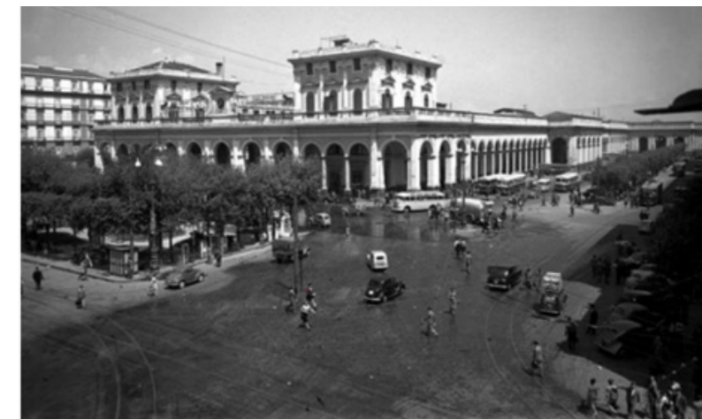
Fig.39 Piazza Garibaldi 1950 before demolition. Taken from Dines, 2012. Photo: Courtesy of AArchivio Fotografico Parisio
