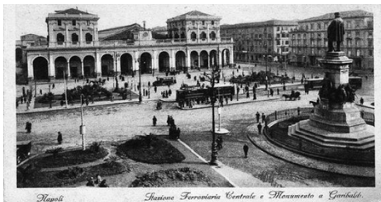
Fig.37 The old Piazza Garibaldi, 1860s. Source: https://i.pinimg.com
