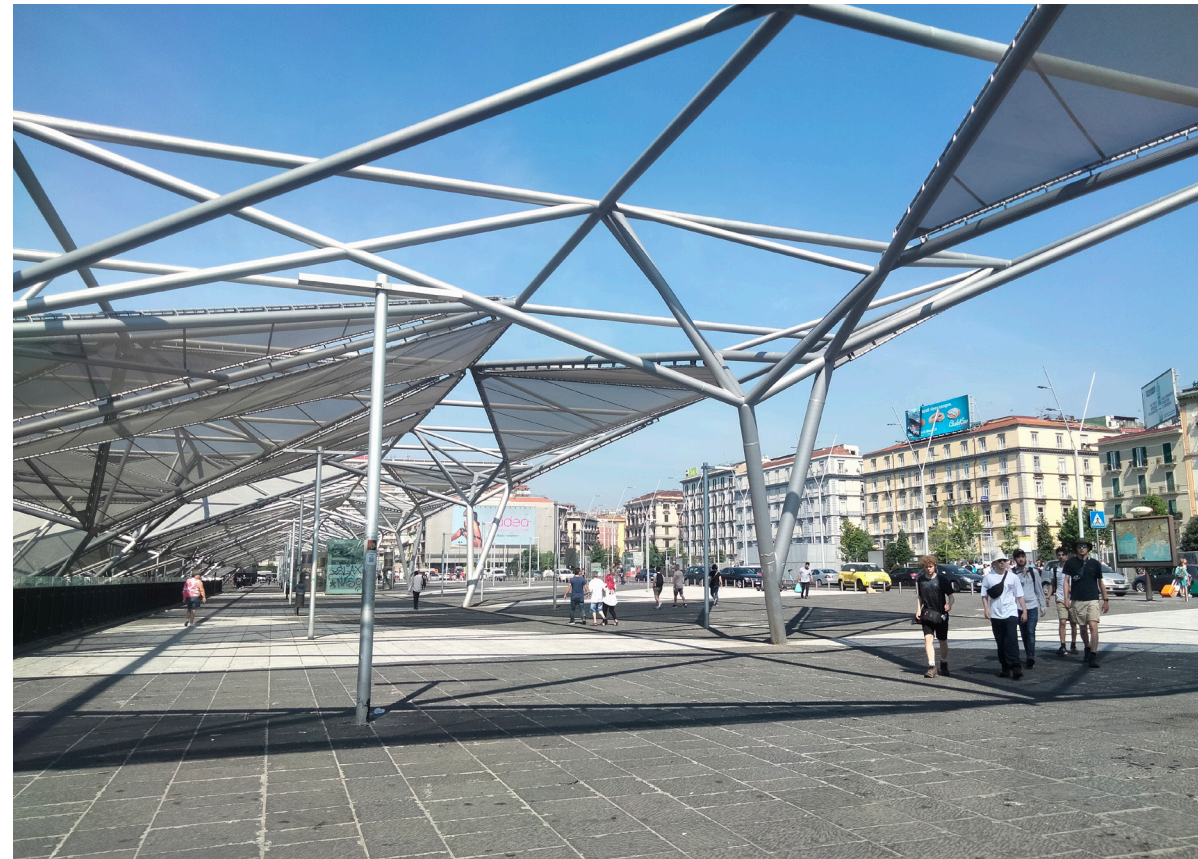
Fig.45 New structure above the new Gallery of Piazza Garibaldi
