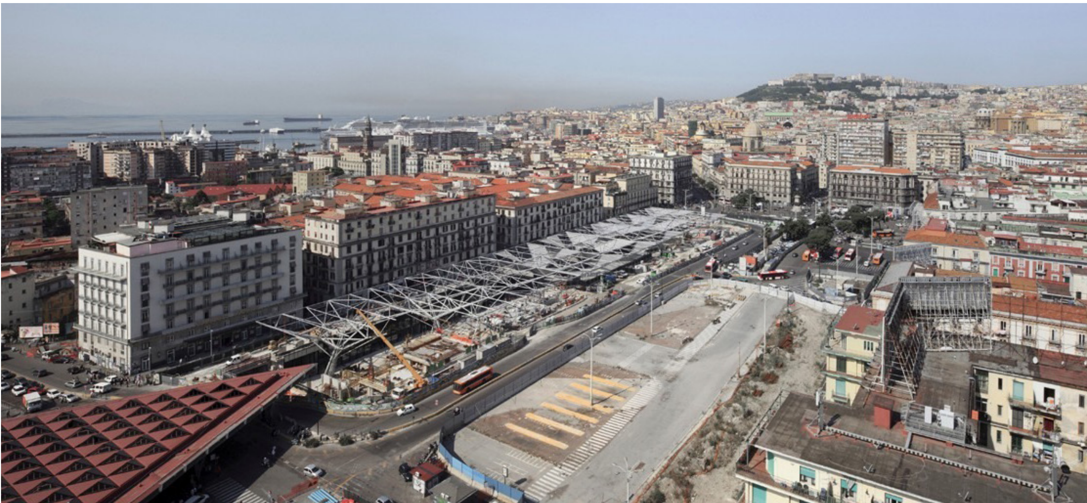
Fig.52 The construction of Piazza Garibaldi in Napoli, retrieved from archilovers.com on 16 July 2023
