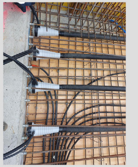
Site photos : These photos represent post tensioning of a slab
