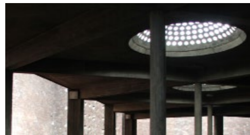
Fig.78 Interior view seeing the cupola.
