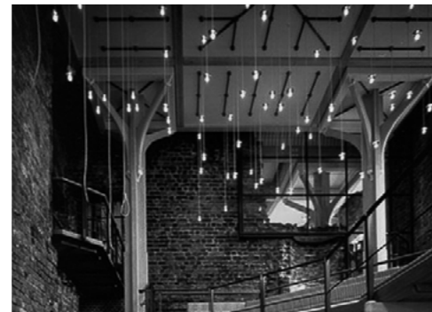
Fig.65 View from interior seeing the material combination and untouched new structure.
