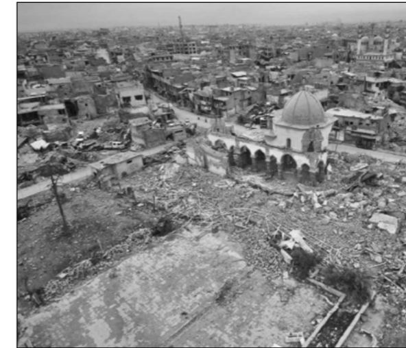
Fig.26 Drone View of Al Nouri Complex after its destruction in 2017.
