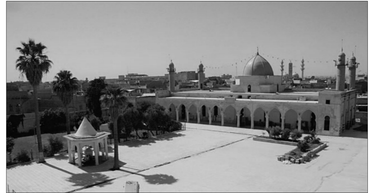
Fig.09 Mosque of al-Nuri. General view of the mosque from the northwest by Petr Justa, 2012.
