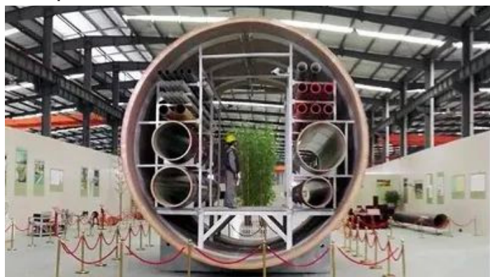
Bamboo winding pipe gallery (33, Jiang Zehui)
