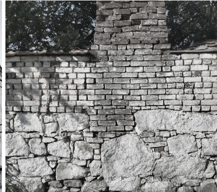
Granite masonry wall and brick
