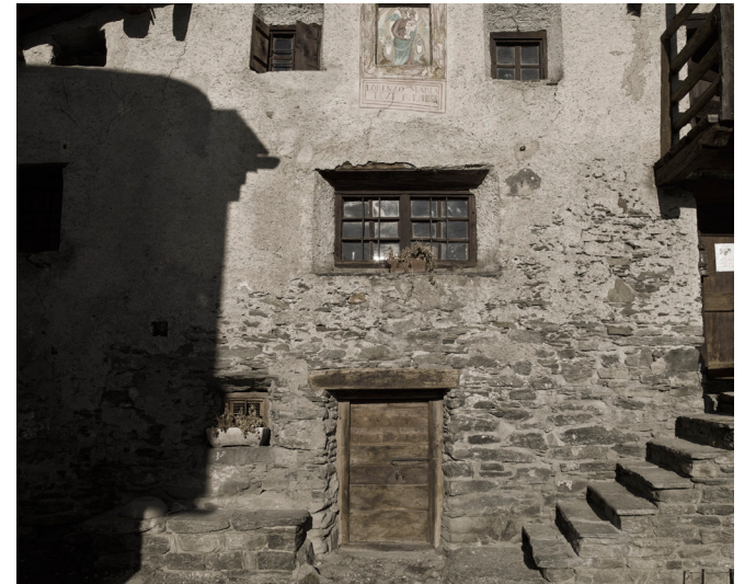
Figure 13- Cà Bardassa facade
