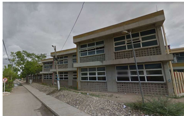
Figure 3-3-2: Outside view of a classroom
