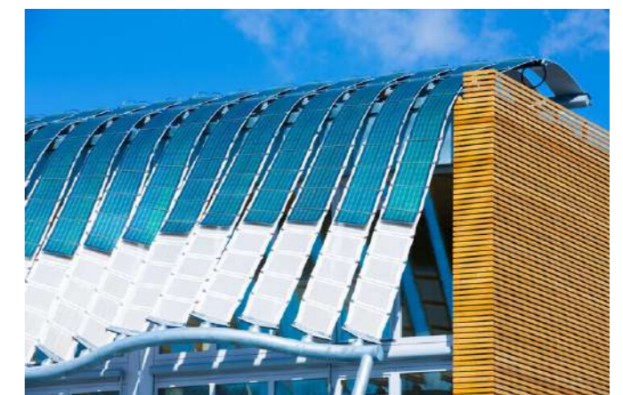
Figure 5.5 Example of thin film solar cell
