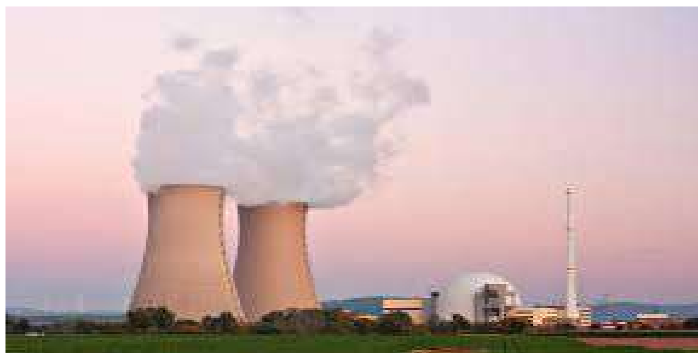
Figure 1.6 Nuclear power plant in Grohnde near Hameln in Lower Saxony, Germany
