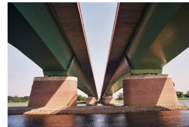
Figure 1.21 Bridge of the A9 near Dessau crossing the river Elbe
