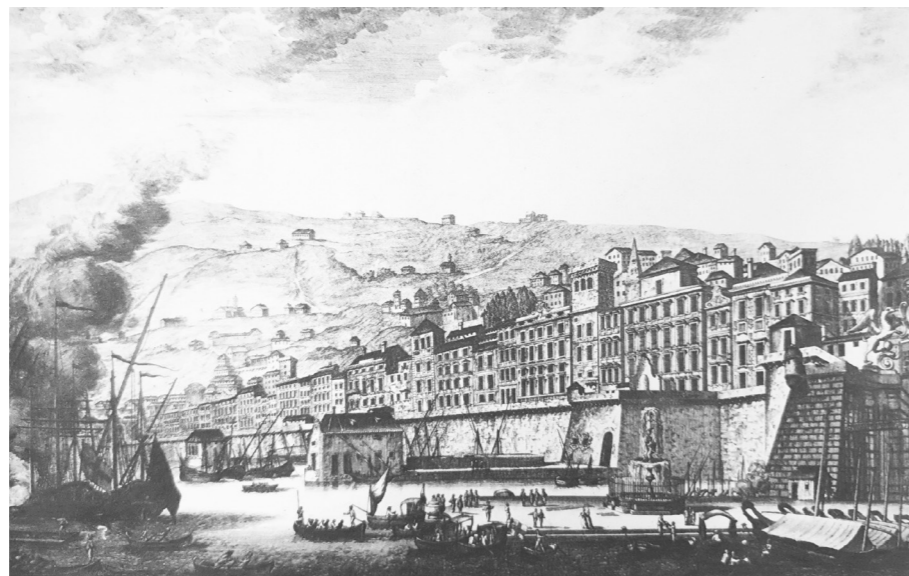
Fig.13. View of the buildings of underpasses with bridges Reale, Spinola e Calvi, leaning against the "sea walls". It represents an example of defensive infrastructure (Poleggi & Cevini, 1981)
