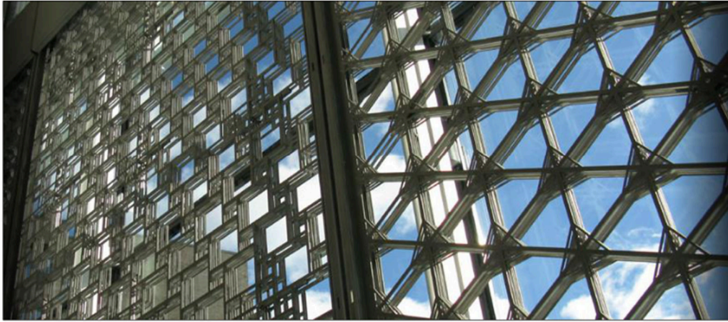
Figure 20: triangular and rectangular Tessellate pattern of Simons center at stony brook university (Jamil Alkhayyat J 2013)
