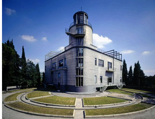
Figure 2: The first building with Kinetic Architecture was Villa Girasole where girasole means sunflower designed by Angelo Invernizzi in 1935, which follows the sun path (Alter 2017).
