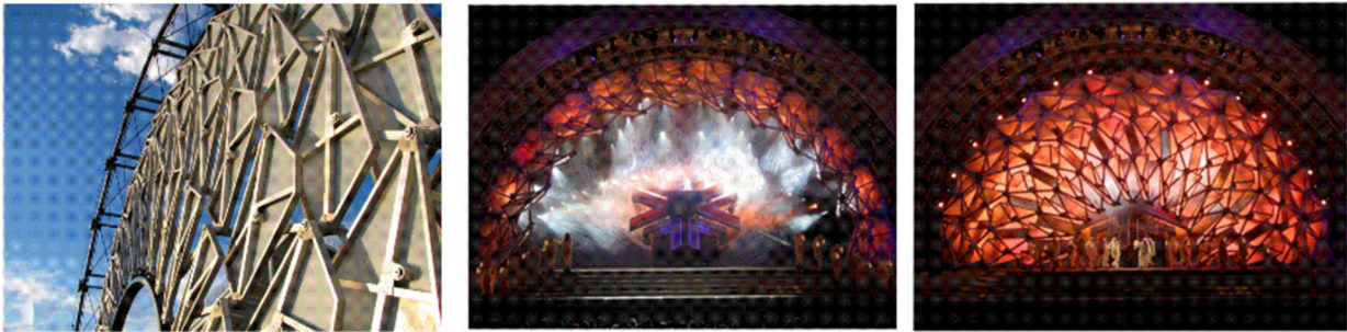
Figure 9: Hoberman Arch , an example of kinetic architectural structure using rigid devices, aluminium profile modules moving by electronic motors (Stevenson 2011).
