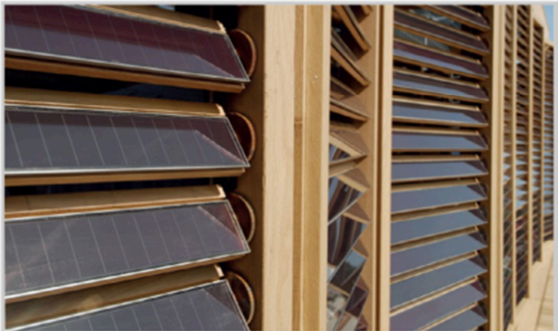
Figure 26: Intelligent facade of automated wood louvers with building integrated Photovoltaics create a continuous facade for TU Darmstadt's 2007 Solar Decathlon House. (Source: Thun and Velikov, 2013)
