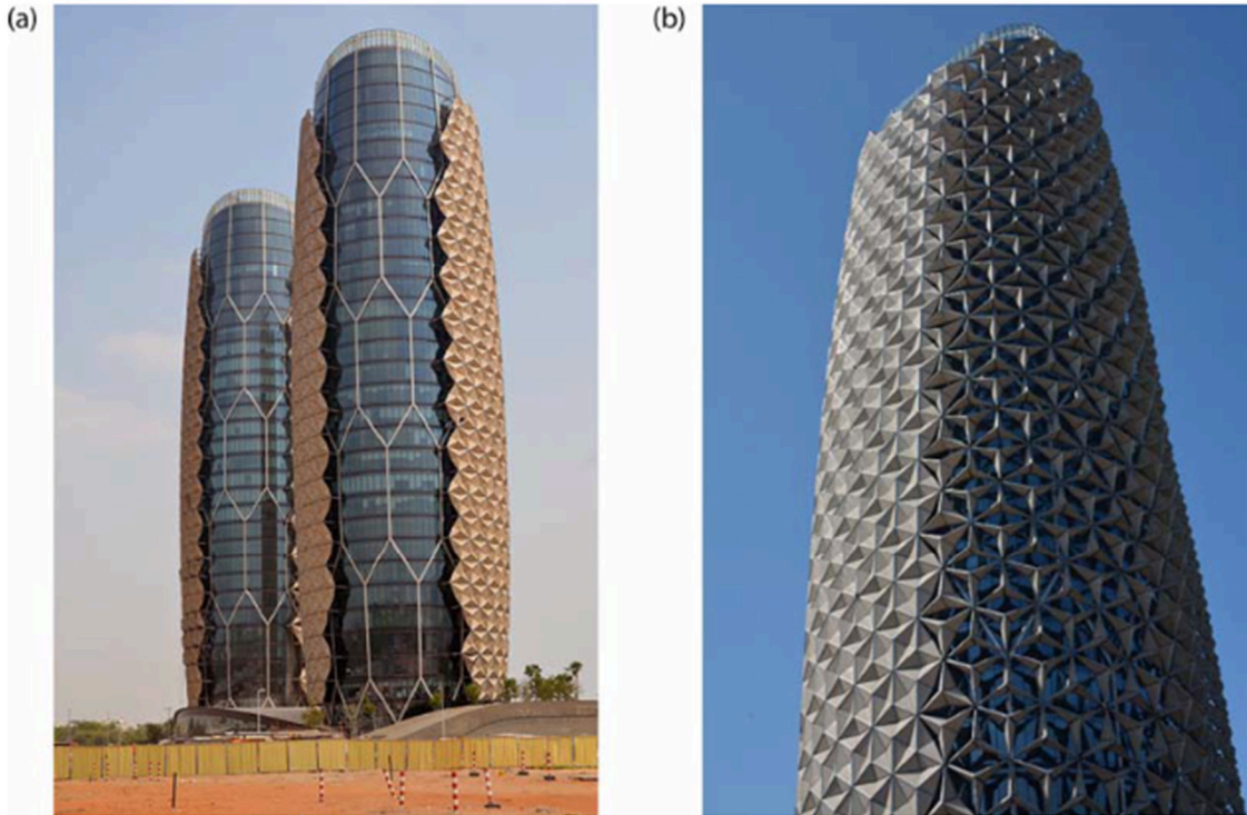
Figure 14: (a) Northern facade and (b) south facade of Al Bahr Towers, with some opened and closed shading devices. coordinates: 24° 27' 23" N, 54° 24' 4" E; alt: 3m (photo courtesy: Terry Boake).
