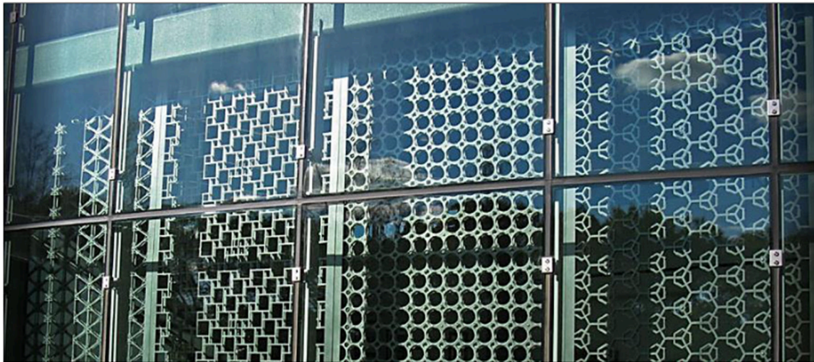
Figure 18 : Tessellate system façade of Simons center at stony brook university (Jamil Alkhayyat J 2013)
