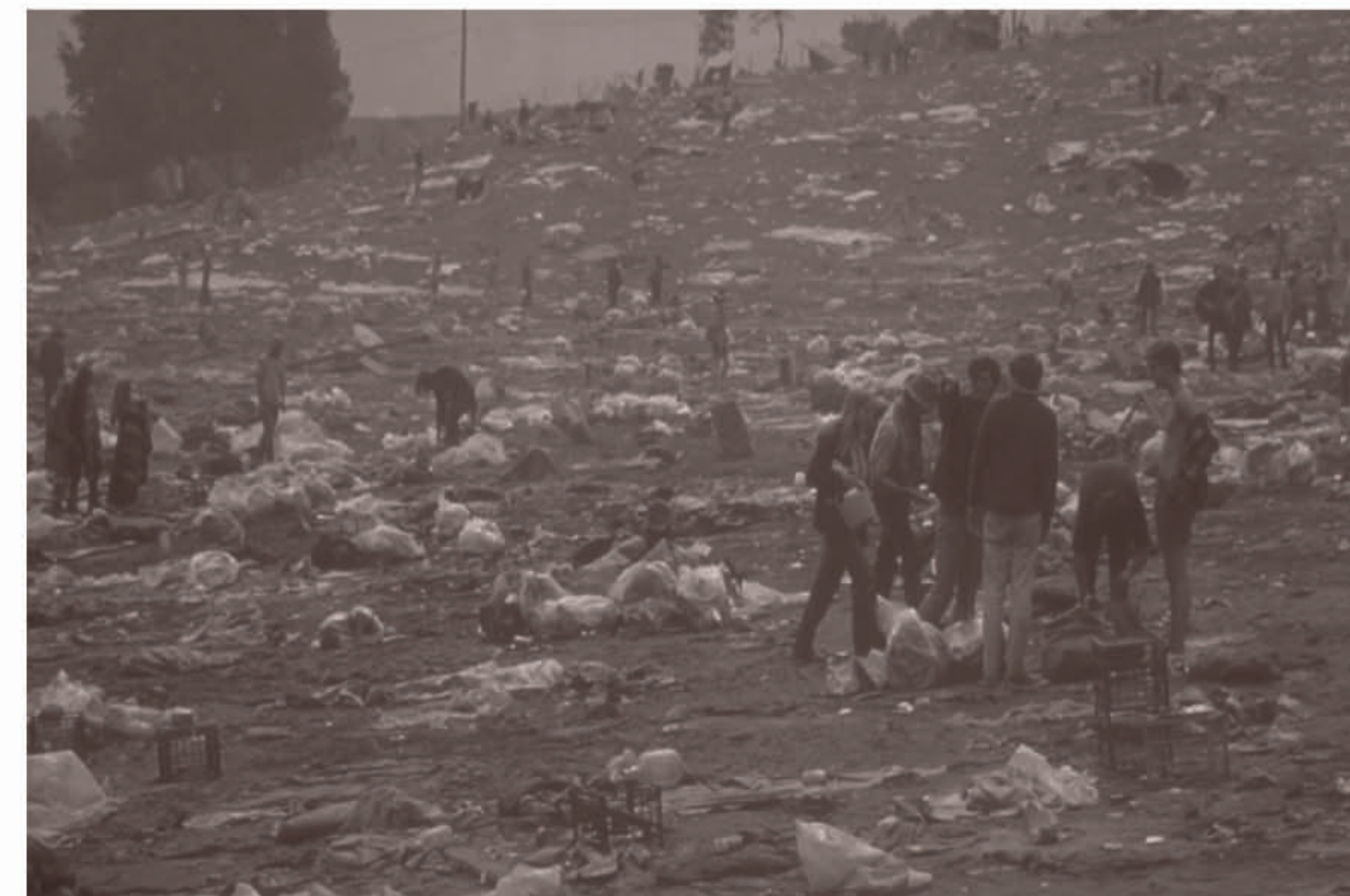
14- Woodstock officially ended on Monday, August 18. After Hendrix left the stage. Cleaning up the venue was a mammoth task and required several days, many bulldozers and tens of thousands of dollars.
