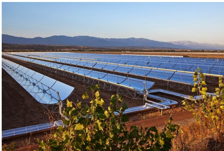
Figure 1-9: Parabolic Trough Plant, CSP Spain Orellana. [14]
