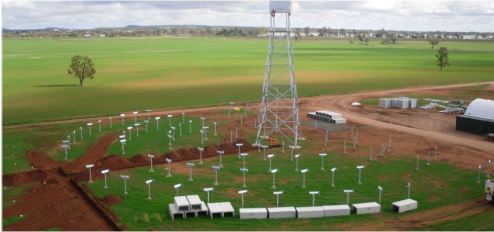
Figure 2-11 One Module of Solastor's Graphite Receiver at Lake Cargelligo During Construction. [32]
