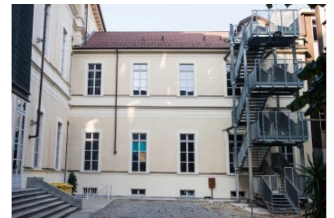
Back of the Building Before Renovation
