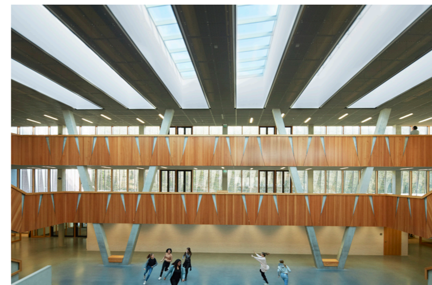
Figure 16. The three-storey atrium of Hessenwald School in Germany. Using six VELUX Modular 'Longlights' to provide optimal daylight conditions.
