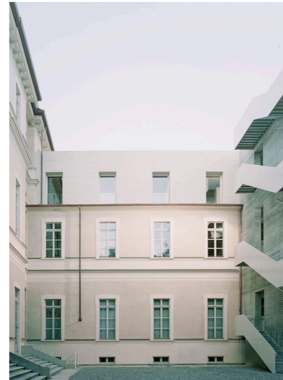
Back of the Building After Renovation
