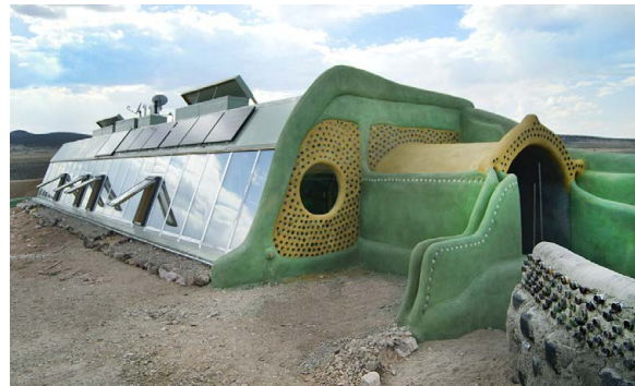
Figure 471. Exterior and interior. Source: Earthship Biotechnology
