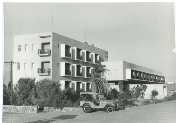
Figure 362. Eilat Hotel (The first hotel in the city), 1967, Source: Eilat's Archive
