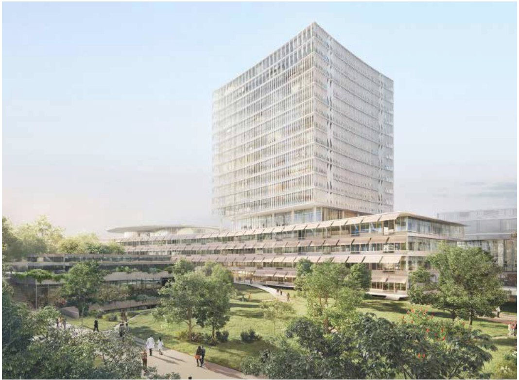
Department of Biosystems Science and Engineering (DBSSE) - ETH Zurich, Nickel & Partners, 2014, (Under Construction)
