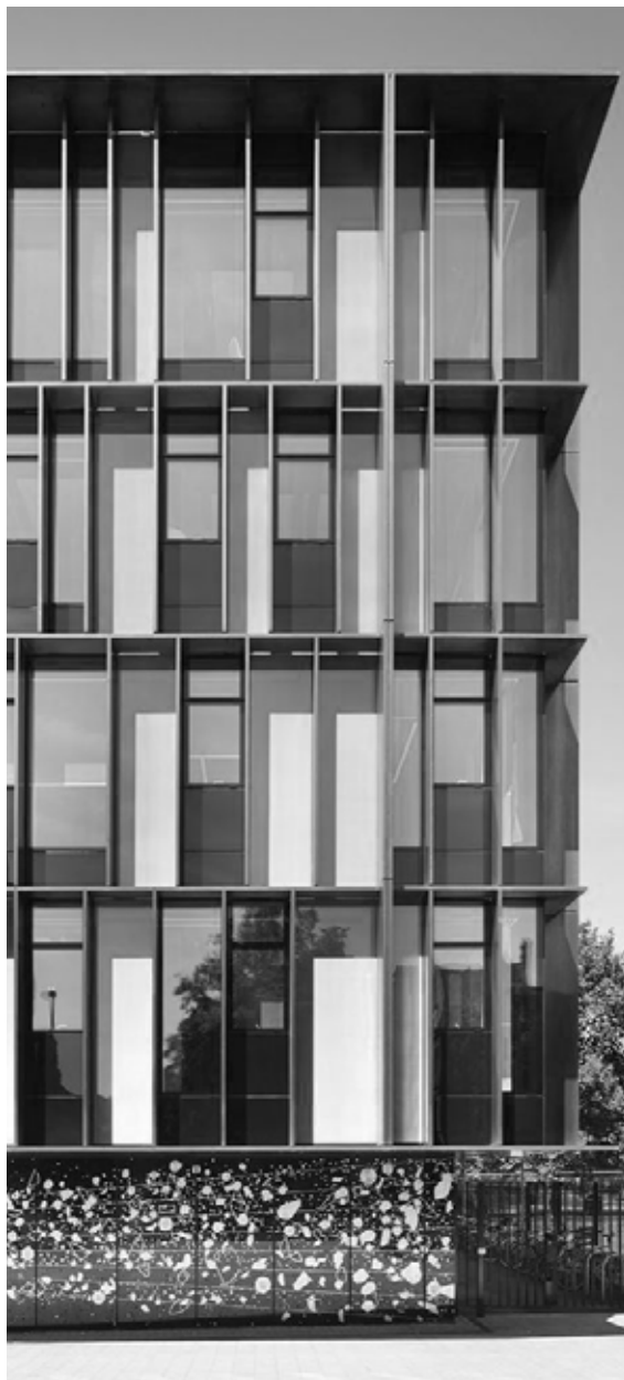
Beecroft Building Hawkins\Brown Architects, Oxford
