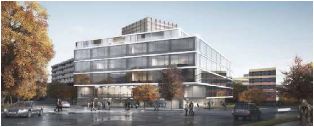
Department of Biosystems Science and Engineering (DBSSE) - ETH Zurich , Nickel & Partners, 2014, ( Under Construction)
