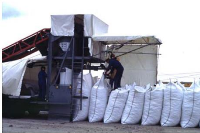
Figure 11. Photograph of filling plant for geosynthetic containers [16]
