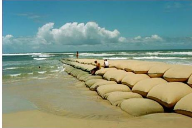
Figure 12. Photograph Sea Groyne with geotextile containers [16]
