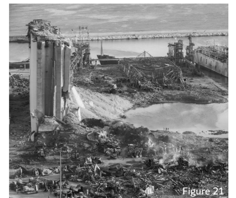
Beirut Port Silos Ruin, 2020
