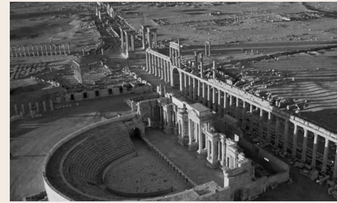
Arcaded street, Palmira.
