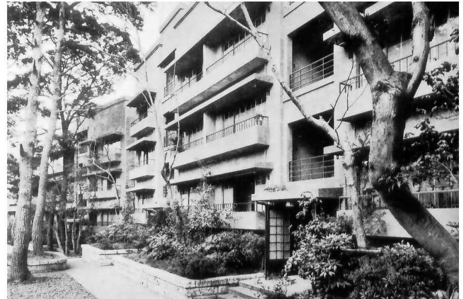
Figure 1.26 Dojunkai Harajuku Apartments, Tokyo (c. 1920s–30s). Source: Wikimedia Commons
