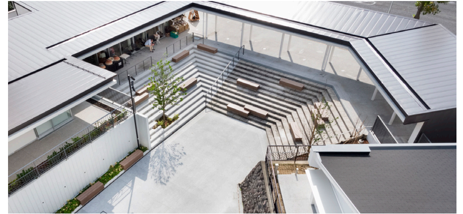
Figure 1.65 Yokodai Sunken Plaza. Photograph by Takumi Ota. Source: Kashiwasato.com
