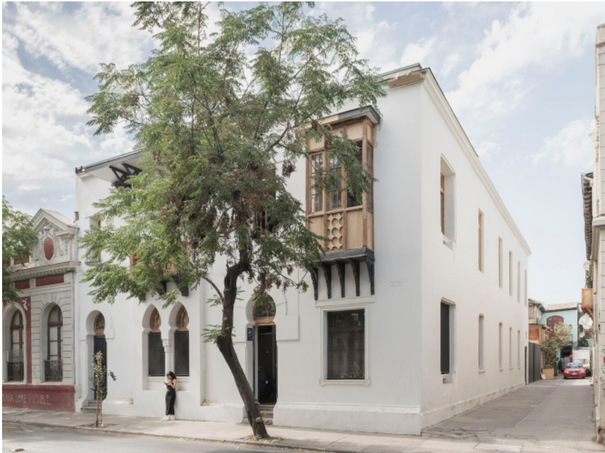
COWORK INTERIORS , Building restoration in Chile
