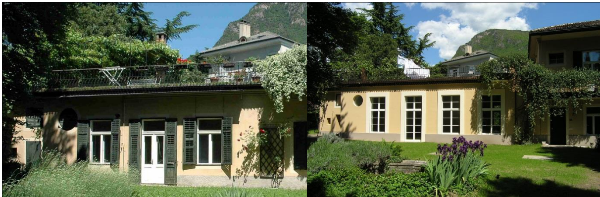
Ansitz Kofler before (2007) and after retrofit
