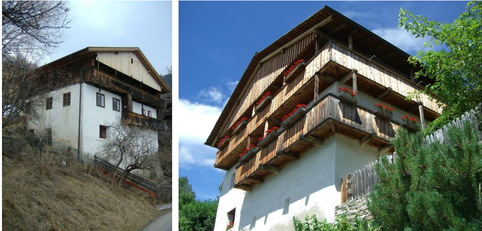
Huberhof/Maso Huber before and after retrofit
