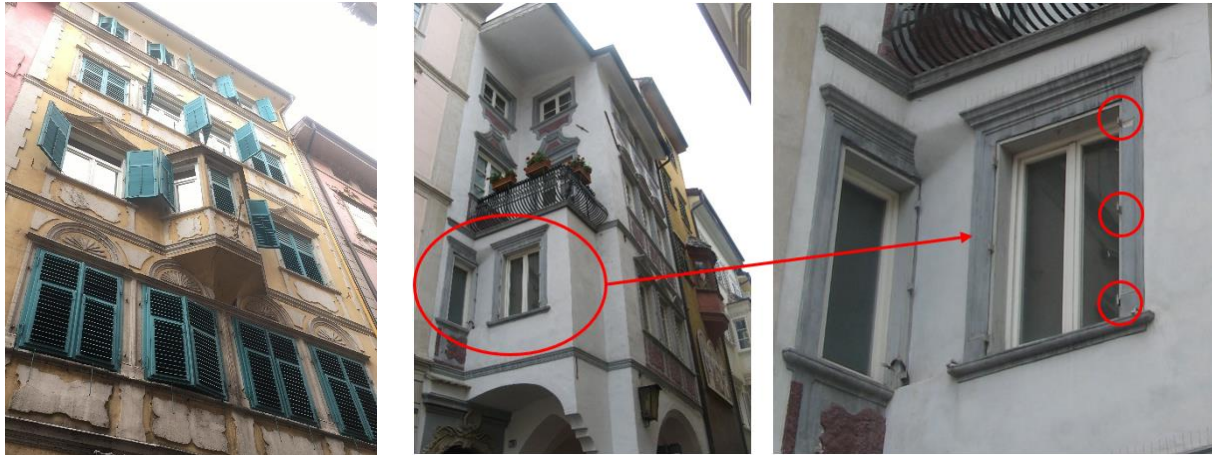
Figure 65 Wooden shutters with orientable slats in Bolzano with Figure 66 The hinges of wooden shutter in Piazza Erbe 11
