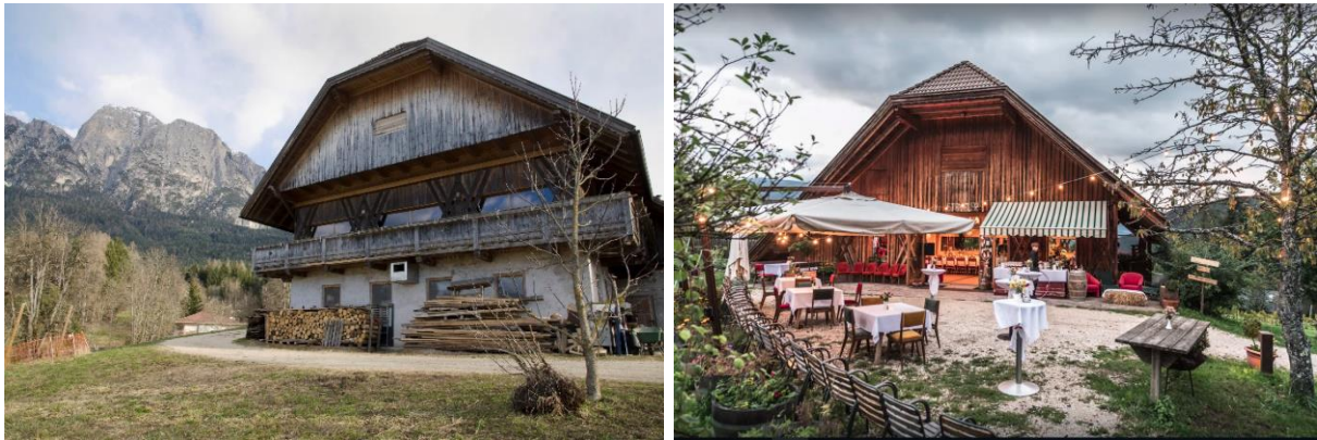
Stanglerhof before and after retrofit
