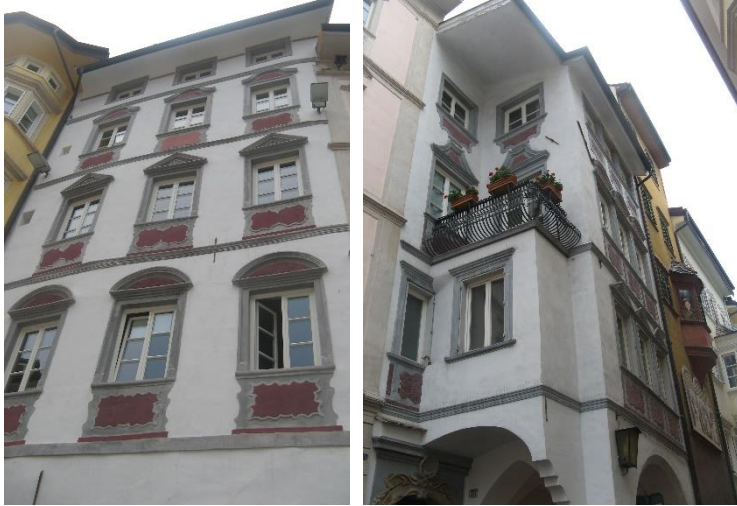
Obstmarkt 11/Piazza Erbe 11 after retrofit
