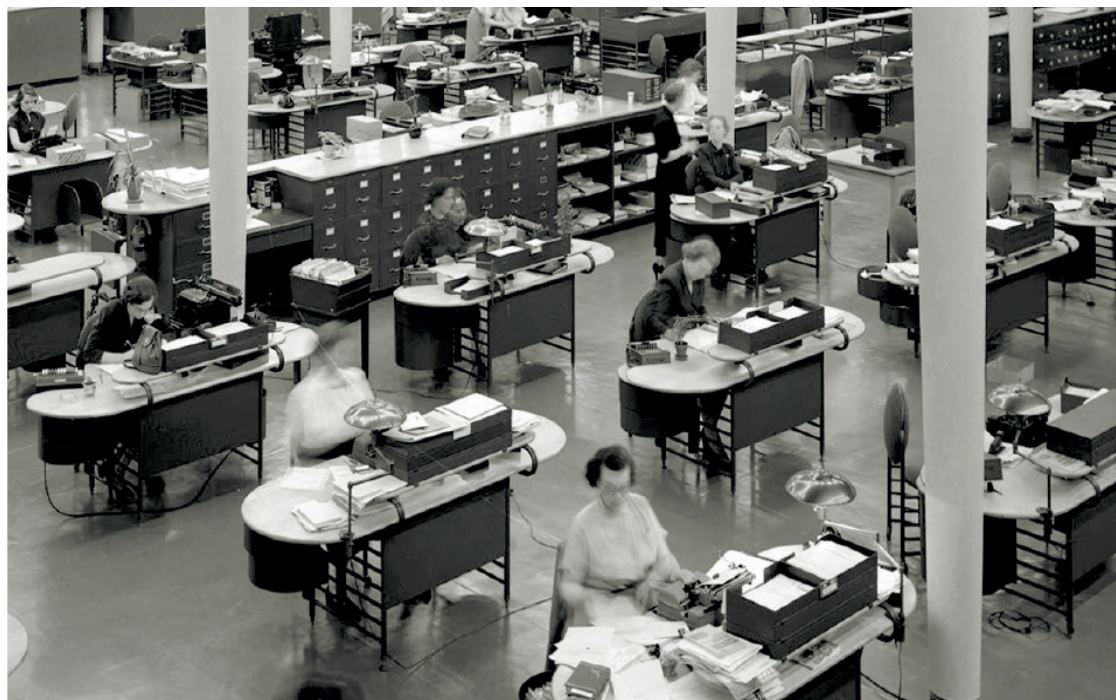
Fig.9 SC Johnson Wax Headquarters by Frank Lloyd Wright, 1936, USA
