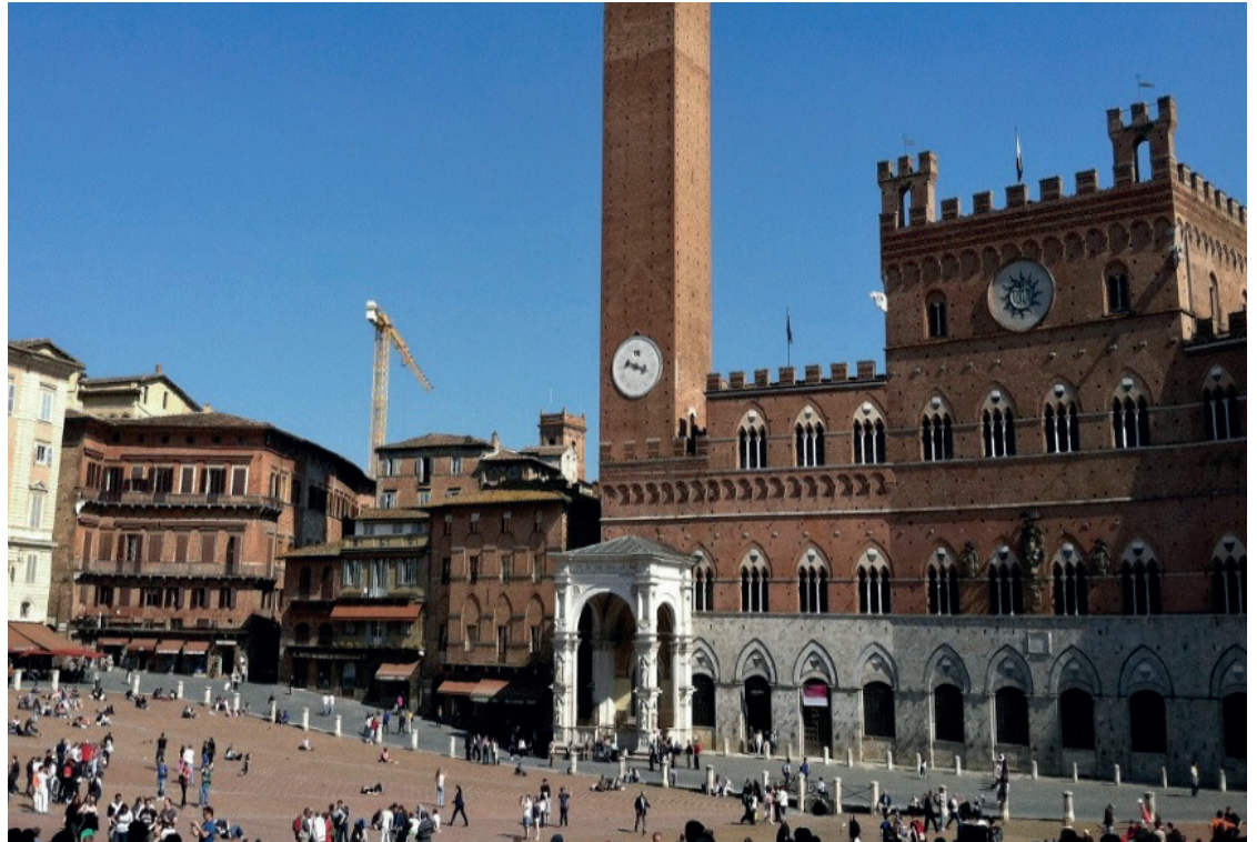
Fig.6 Clock/Bell Tower at Del Campo Square in Sienna
