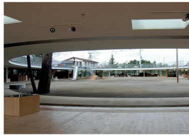
Fuji Kindergarten Tezuka Architects, 2007
