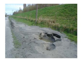
Figure 1.4. Large "sand boil" at the base of the landside of the levee on Coutts Island Road, New Zealand (Green and Cubrinovski 2010)
