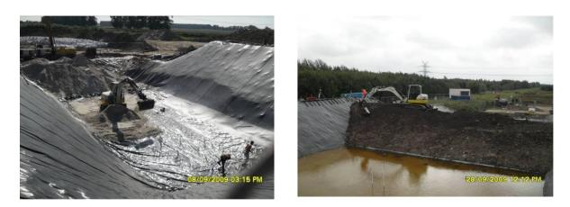
Figure 2.18. Filling of the basin with sand and construction of the levee (Van Beek, Knoeff, et al. 2011)
