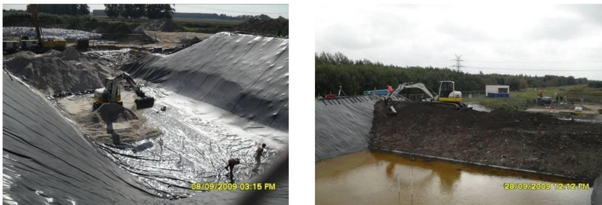
Figure 2.18. Filling of the basin with sand and construction of the levee (Van Beek, Knoeff, et al. 2011)
