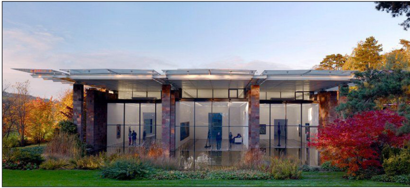
Fig 132/ Fondation Beyeler, Basel by Renzo Piano, Theme of curtain walling and external bonding
