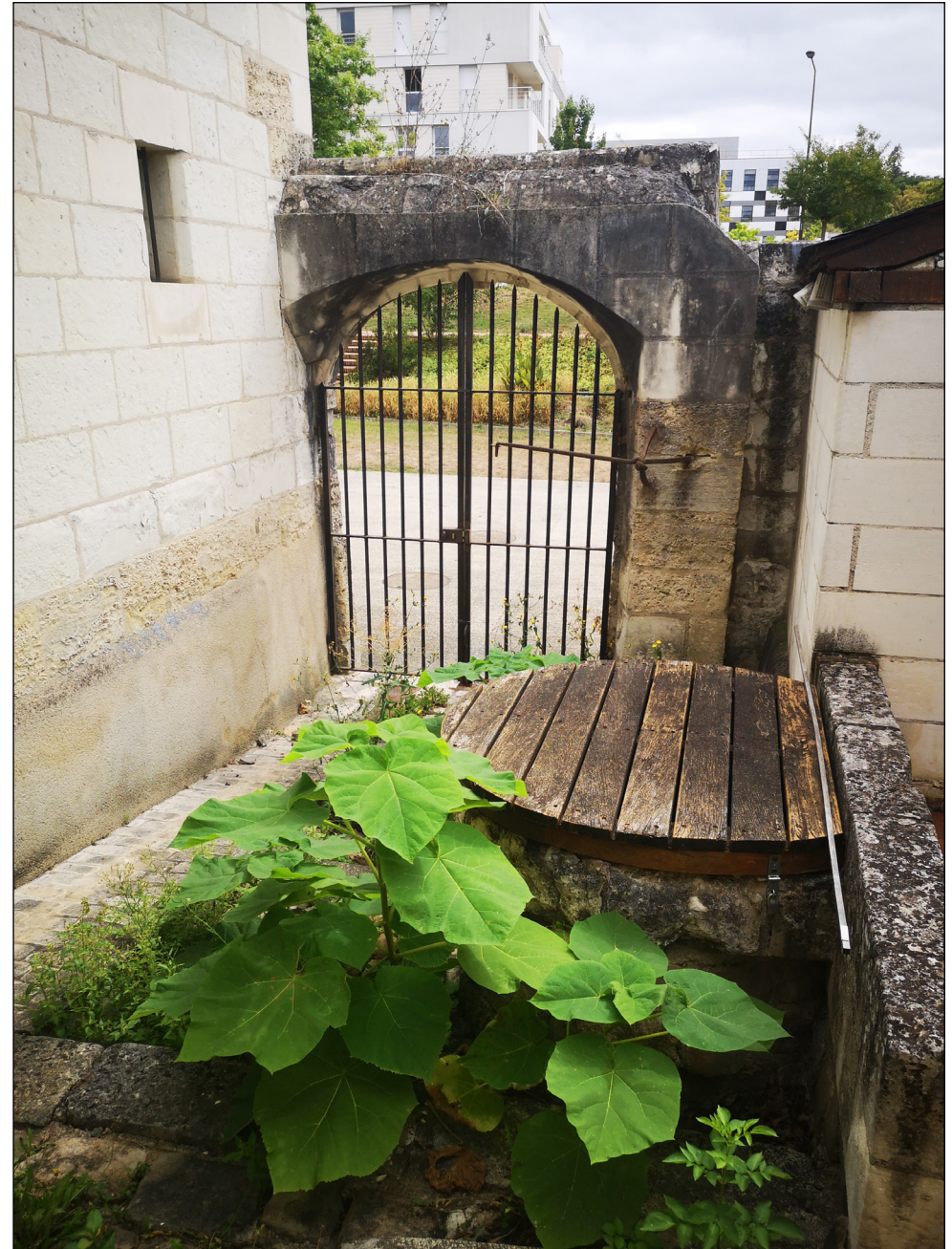
Photographic Database | Subject : View on the gate inside the courtyard PD.06 | Date : 23/08/2022 N°25 | Camera : Huawei P20 (DPI. 429 ppp)
