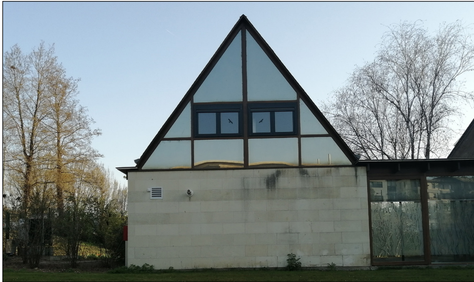
Photographic Database | Subject : View on the north facade of building B PD.03 | Date : 22/03/2022 N°11 | Camera : Huawei P20 (DPI. 429 ppp)
