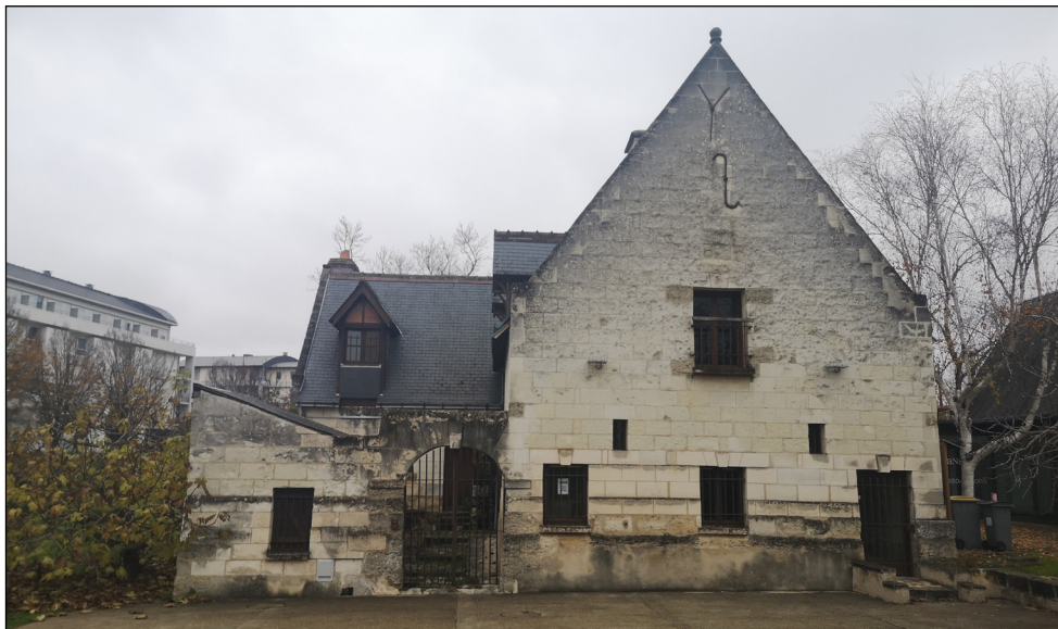
Photographic Database | Subject : View on the south facade of building A PD.02 | Date : 30/11/2022 N°07 | Camera : Huawei P20 (DPI. 429 ppp)
