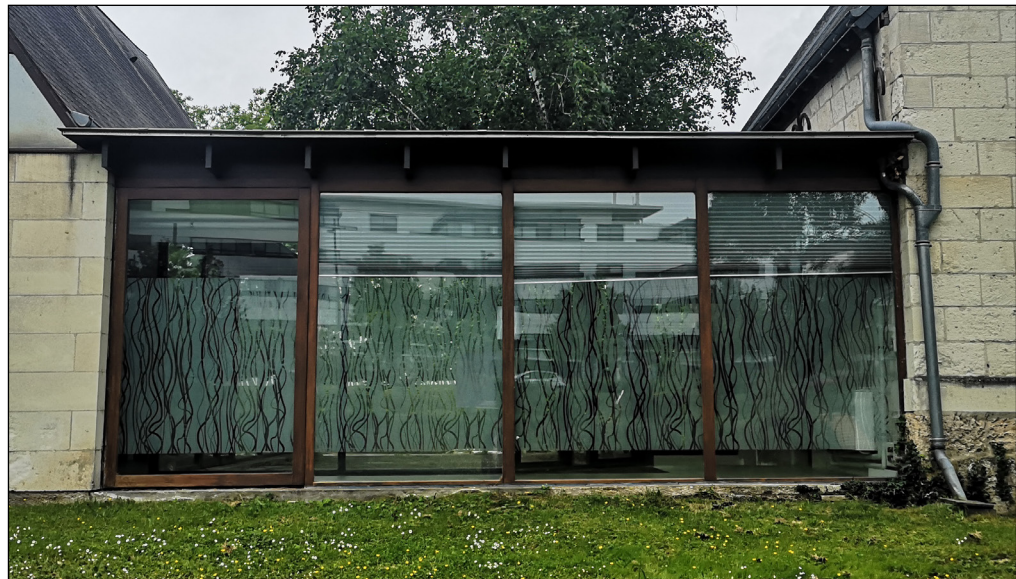
Photographic Database | Subject : View on the north facade of the glasshouse PD.05 | Date : 23/05/2023 N°19 | Camera : Huawei P20 (DPI. 429 ppp)
