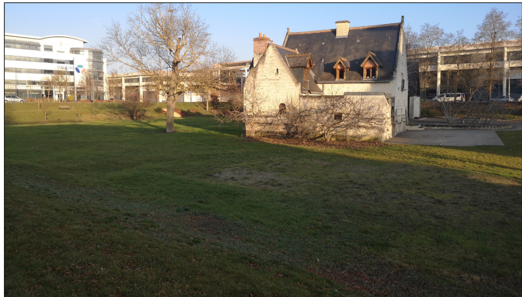
Photographic Database | Subject : View on the west facade of building C PD.04 | Date : 22/12/2021 N°15 | Camera : Huawei P20 (DPI. 429 ppp)
