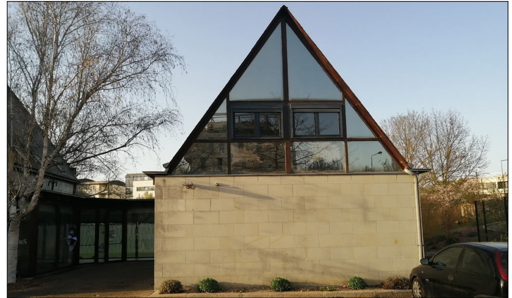
Photographic Database | Subject : View on the south facade of building B PD.03 | Date : 22/03/2022 N°12 | Camera : Huawei P20 (DPI. 429 ppp)
