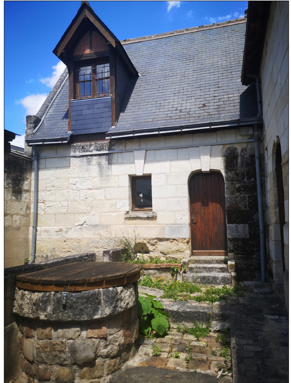
Photographic Database | Subject : View on the south facade of building C PD.04 | Date : 30/11/2022 N°18 | Camera : Huawei P20 (DPI. 429 ppp)
