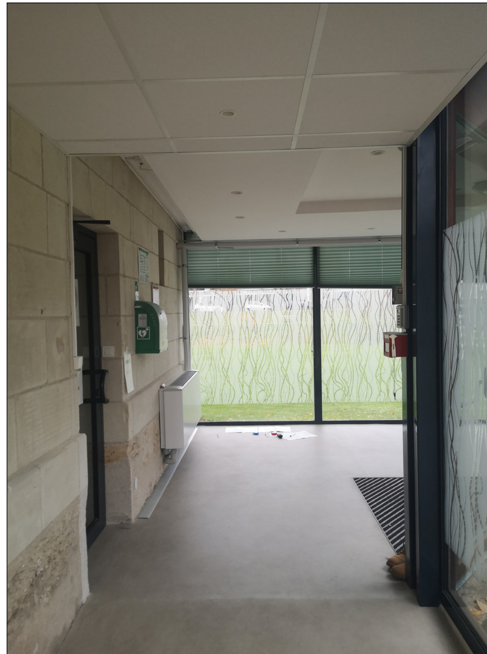
Photographic Database | Subject : View on the entrance (Building A / glasshouse) PD.05 | Date : 30/11/2022 N°22 | Camera : Huawei P20 (DPI. 429 ppp)
