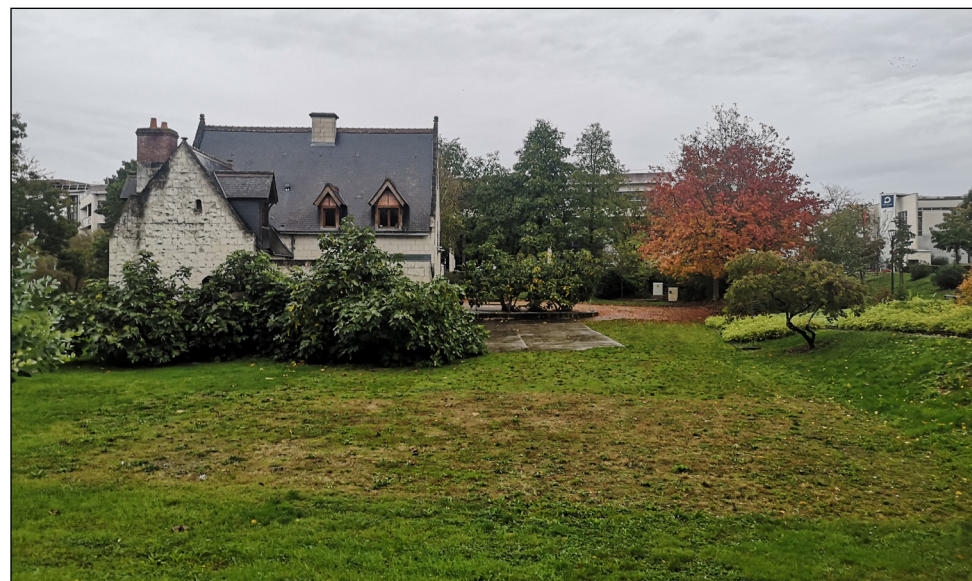
Photographic Database | Subject : View on the farmhouse (from west) PD.01 | Date : 28/10/2023 N°05 | Camera : Huawei P20 (DPI. 429 ppp)
