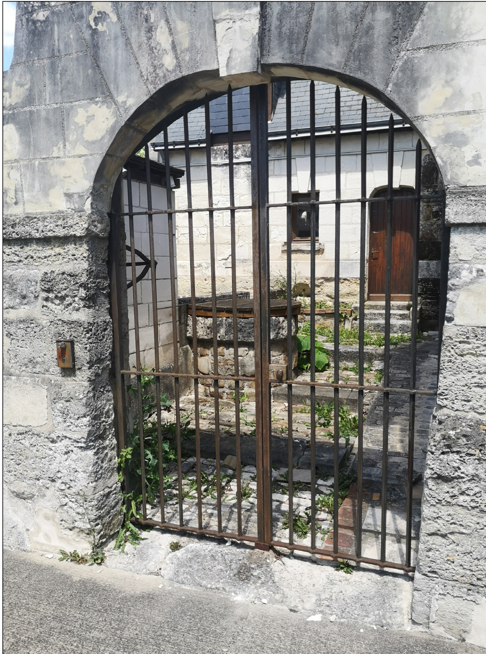
Photographic Database | Subject : View on the gate outside the courtyard PD.06 | Date : 10/06/2022 N°24 | Camera : Huawei P20 (DPI. 429 ppp)
