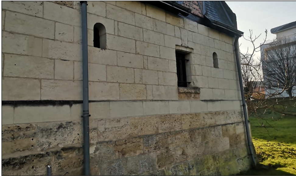
Photographic Database | Subject : View on the north facade of building C PD.04 | Date : 22/12/2021 N°16 | Camera : Huawei P20 (DPI. 429 ppp)
