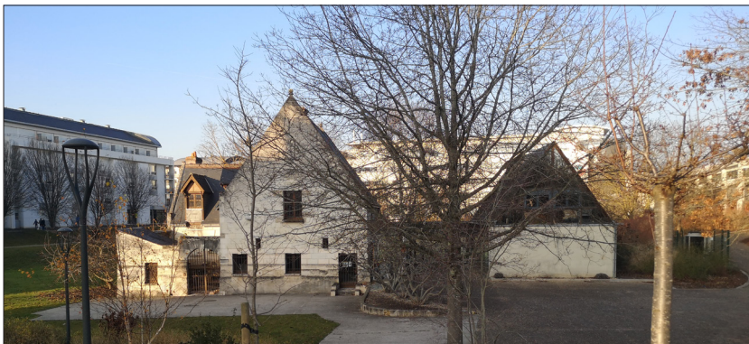
Fig 050/ Current state of the farmhouse from South (photos taken on 30/11/2022)
