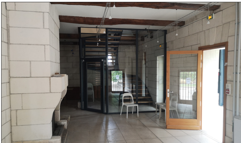
Photographic Database | Subject : View on the main room of building A groundfloor PD.02 | Date : 23/08/2022 N°08 | Camera : Huawei P20 (DPI. 429 ppp)
