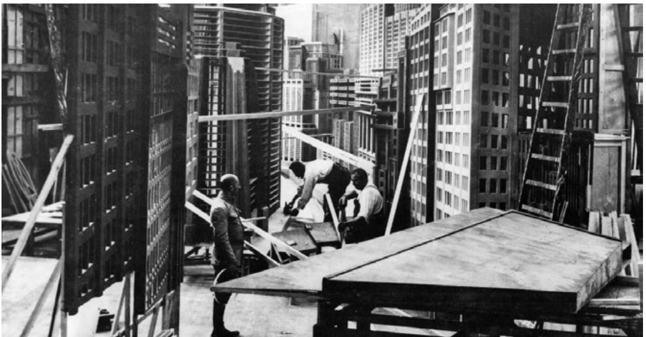
Figure 2. Constructing the set of the City of the Future for Metropolis (1927). Source: Cinema Scholars. Workers building the miniature sets used in Metropolis.
