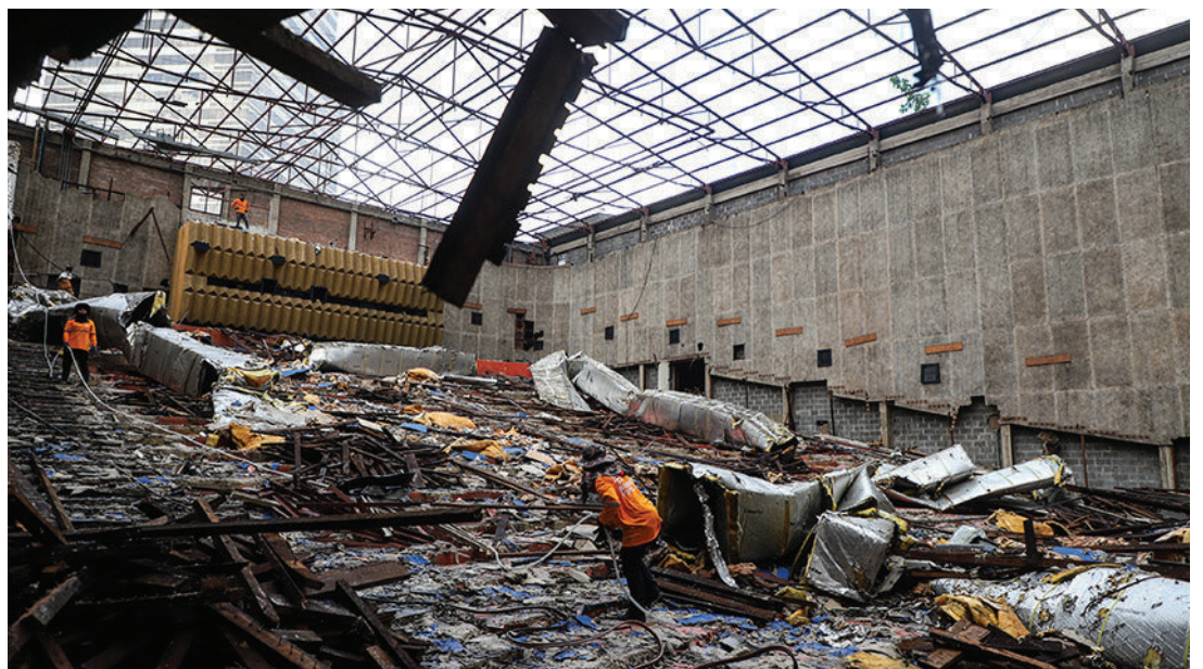
Demolition of Scala Cinema
