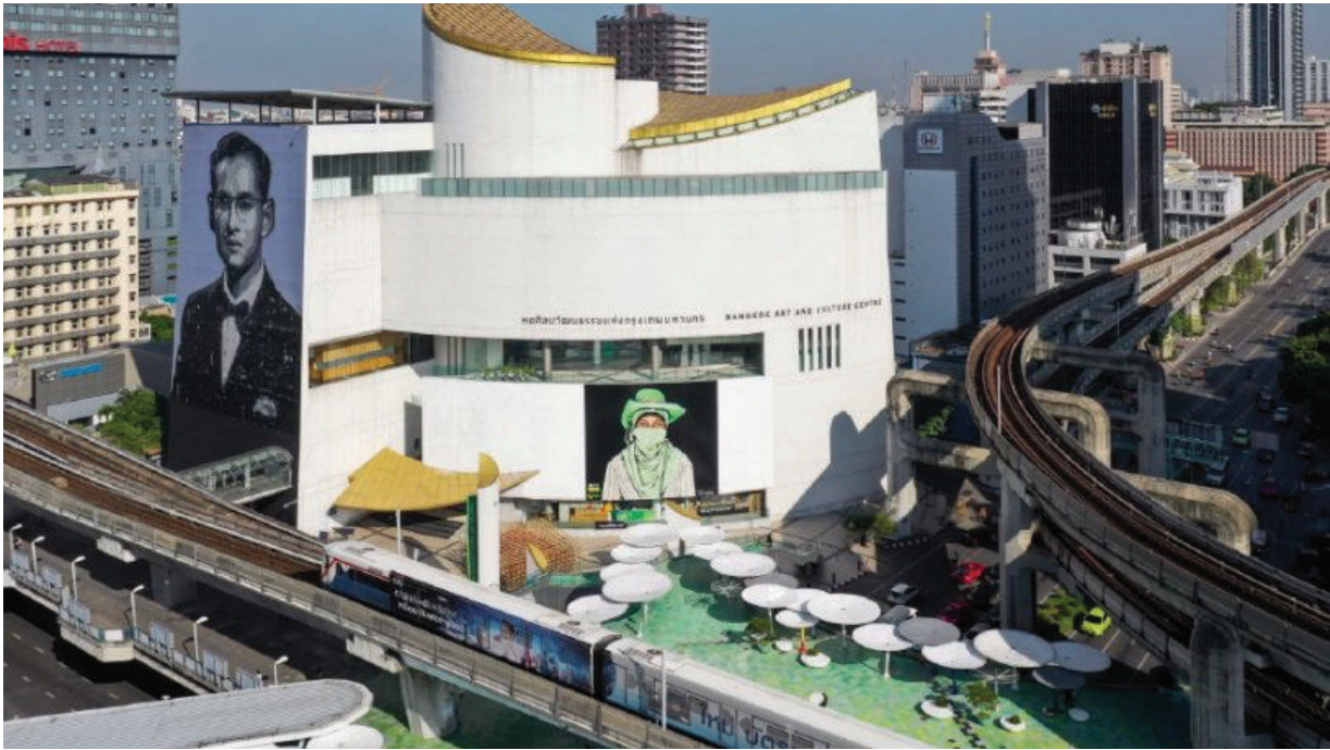
BACC with Skywalk intersection
