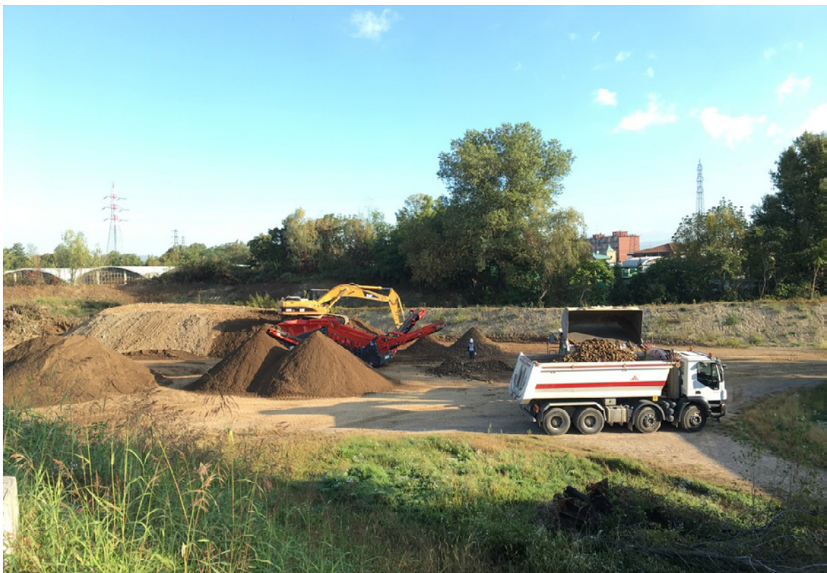
IMAGE_138 _View Of The Sand Embankment Area
