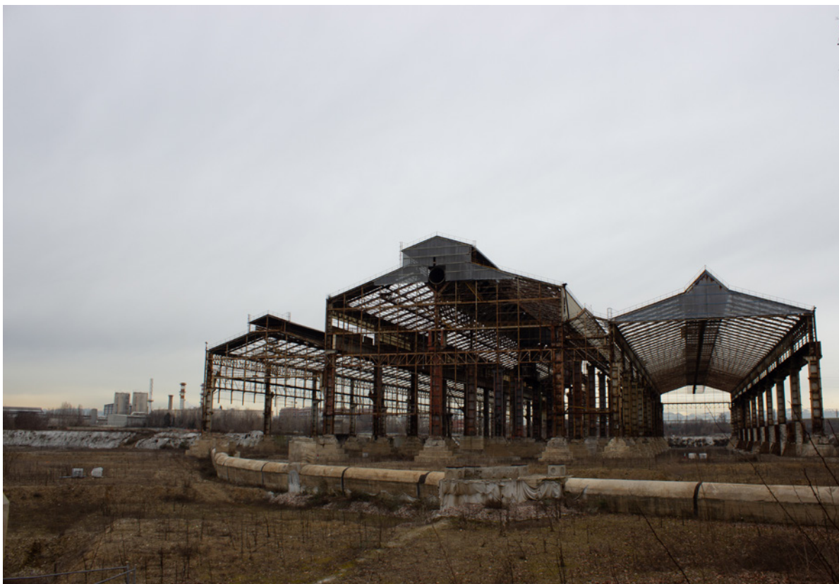
IMAGE_69_T5 Building In The Area Falck
