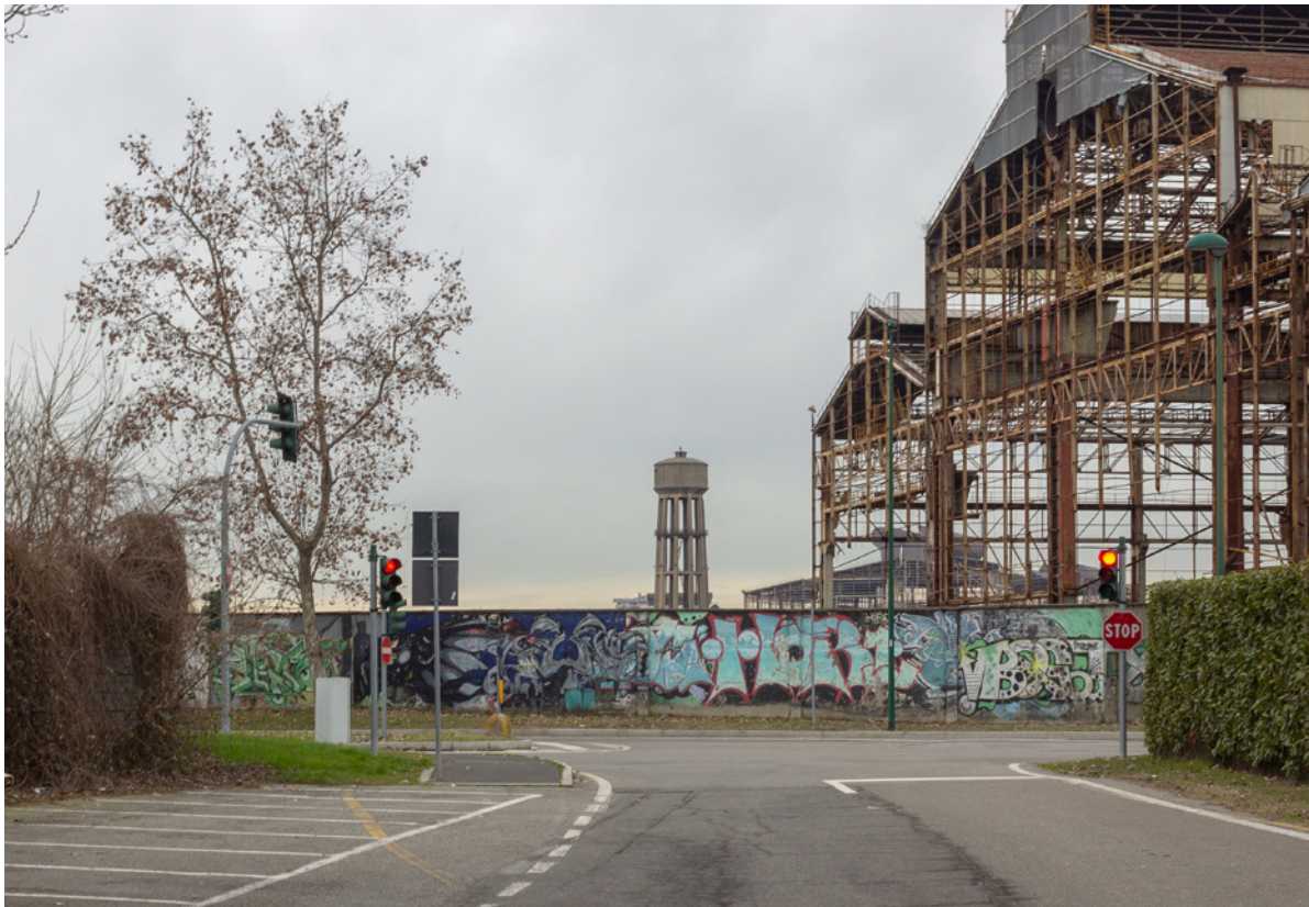
IMAGE_123 Current Situation With No Sidewalks On Via Parpagliona
