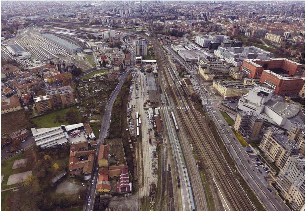
IMAGE_213 _Aerial View Of The Scalo Greco - Pirelli
