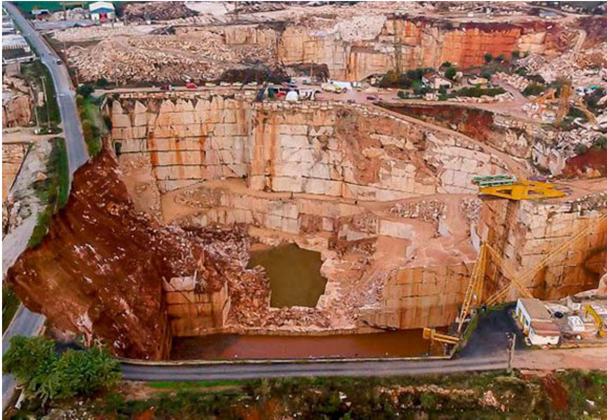
IMAGE_51 _Quarry Collapse In Borba, Portugal (2018)
