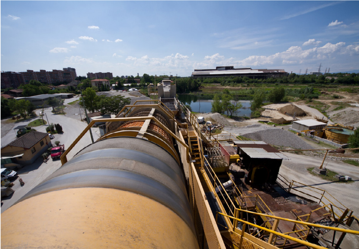
IMAGE_139_Aggregate Processing On The Melzi Quarry
