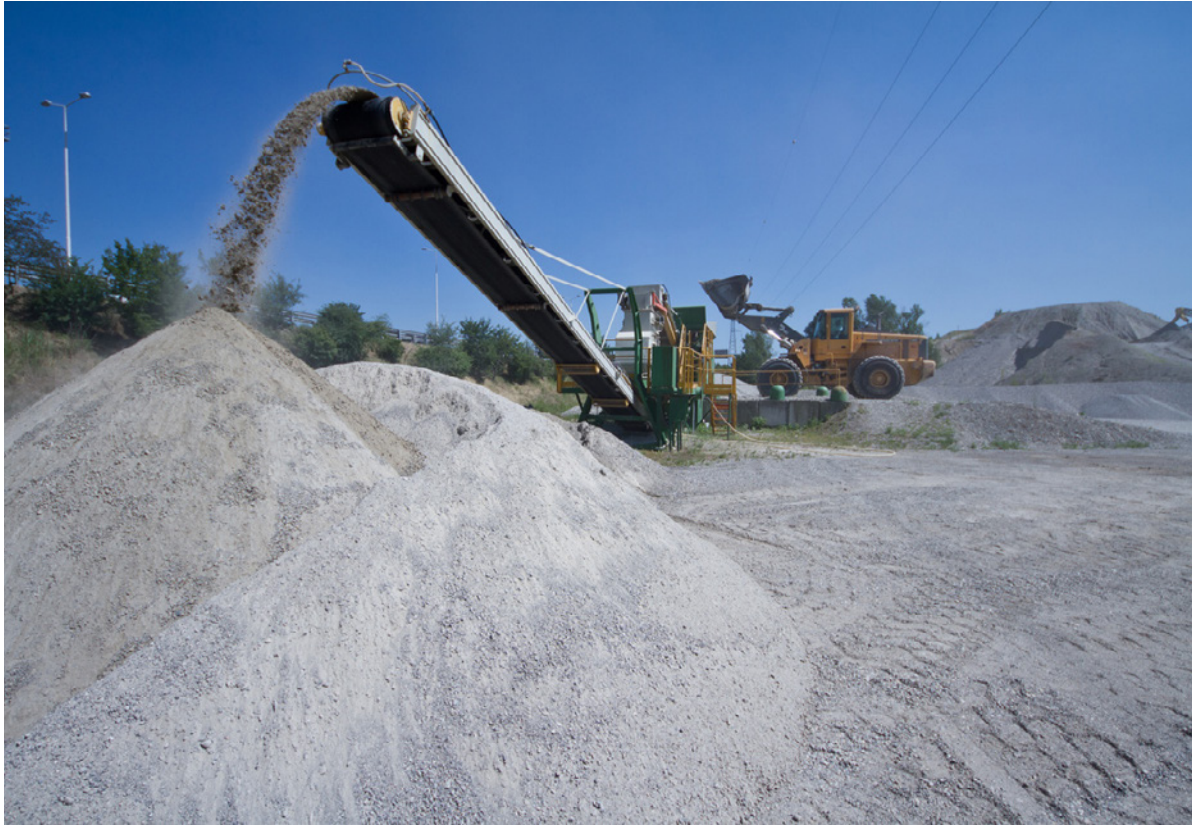
IMAGE_141_ View Of The Concrete Packaging Area
